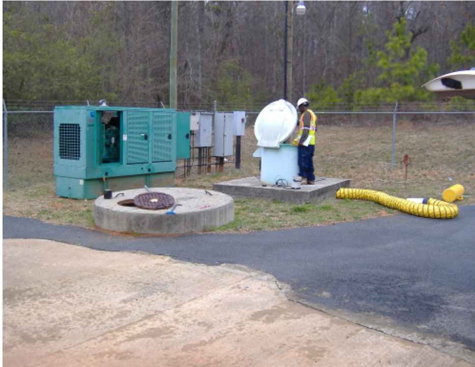
Belowground Lift Station Station and 100-kW Standby Generator
