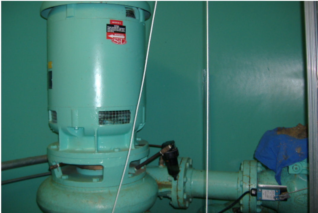
Belowground Smith and Loveless (model: 4D3) 40-hp centrifugal pump (one of two)
