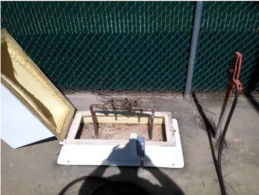
RPZ, HOT BOX, WATER HYDRANT
