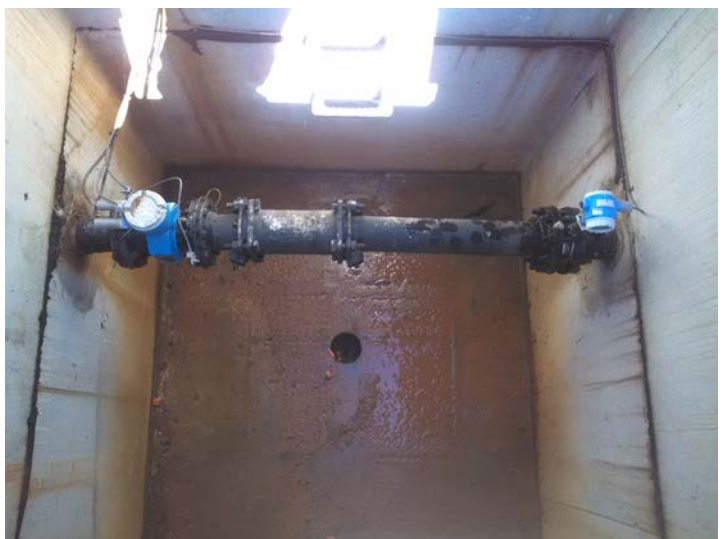
Flow Meter Vault
