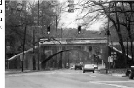
Railroad underpass on Ponce de Leon Avenue.
