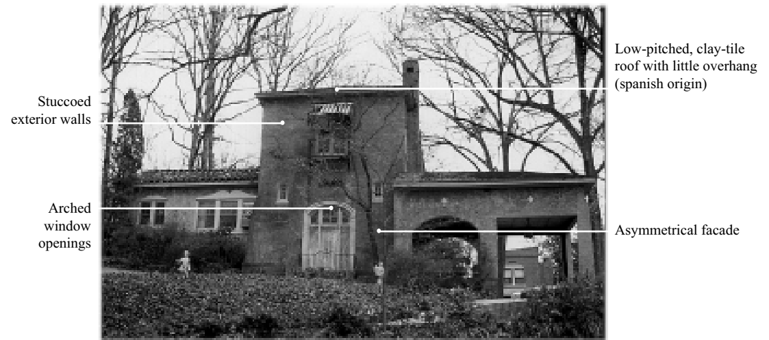
Typical example of the Mediterranean Revival style with principal features keyed.
