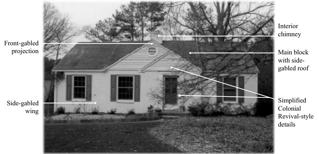
Example of the Emory Grove House Type with principal features keyed.
