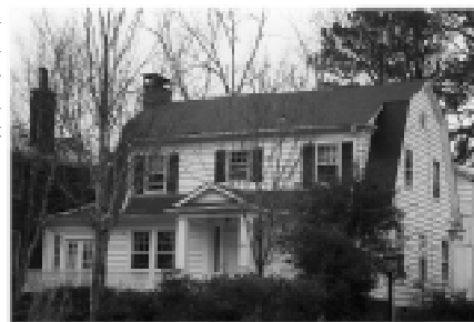
Typical Dutch Colonial Revival House with side-gabled gambrel roof and front shed dormer.
