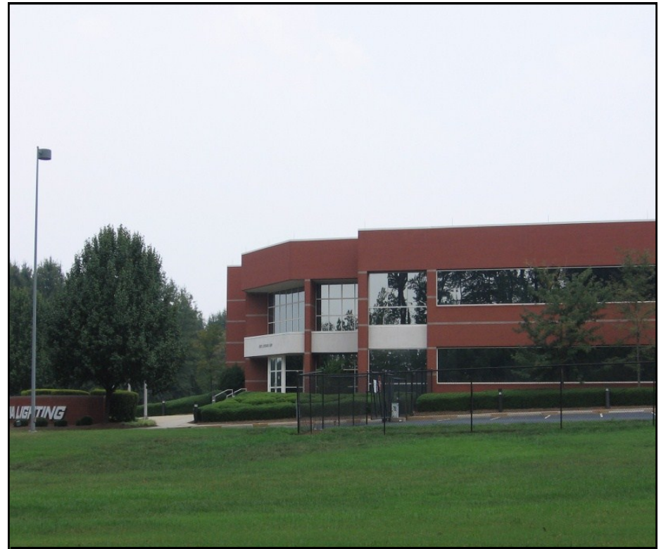
Typical office/distribution building.
