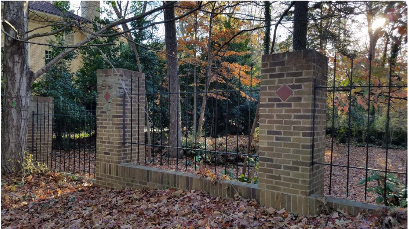
The existing brick and metal fence.
