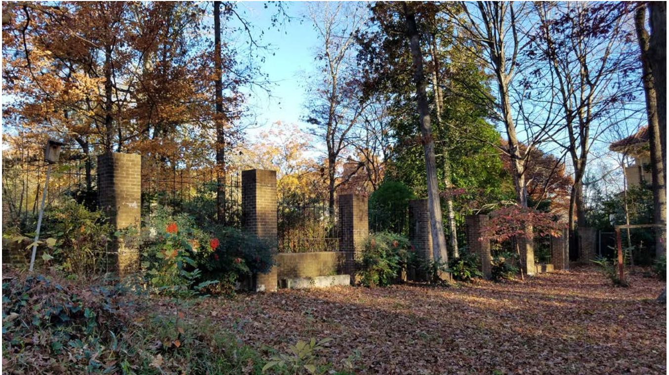
The existing brick and metal fence.
