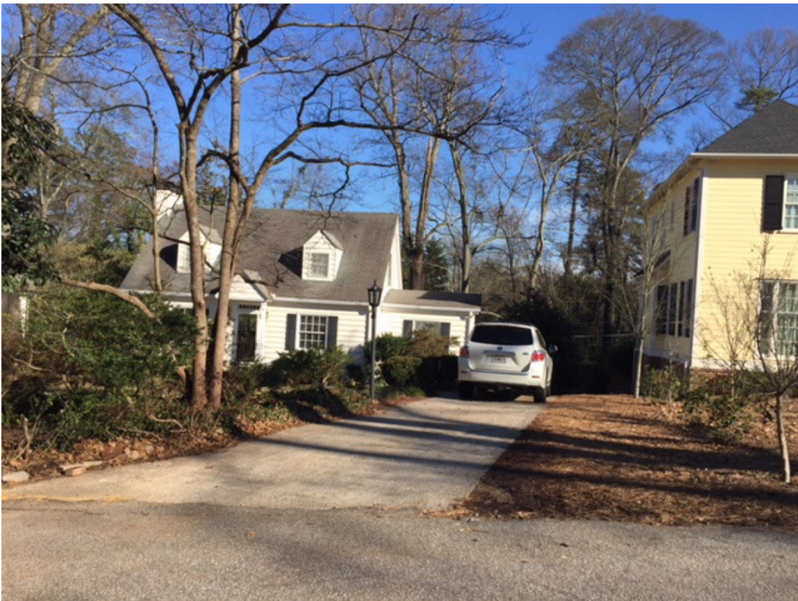
View of Front of House from ROW
