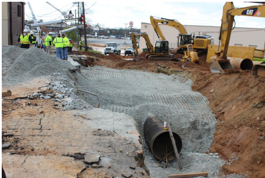
A boil water advisory has been cancelled after crews repair a broken water main.
