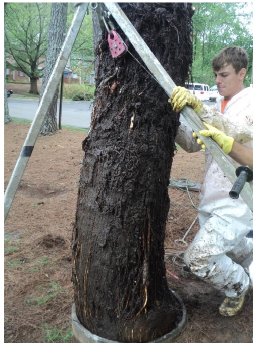
Workers remove a massive root from a sewer line.
