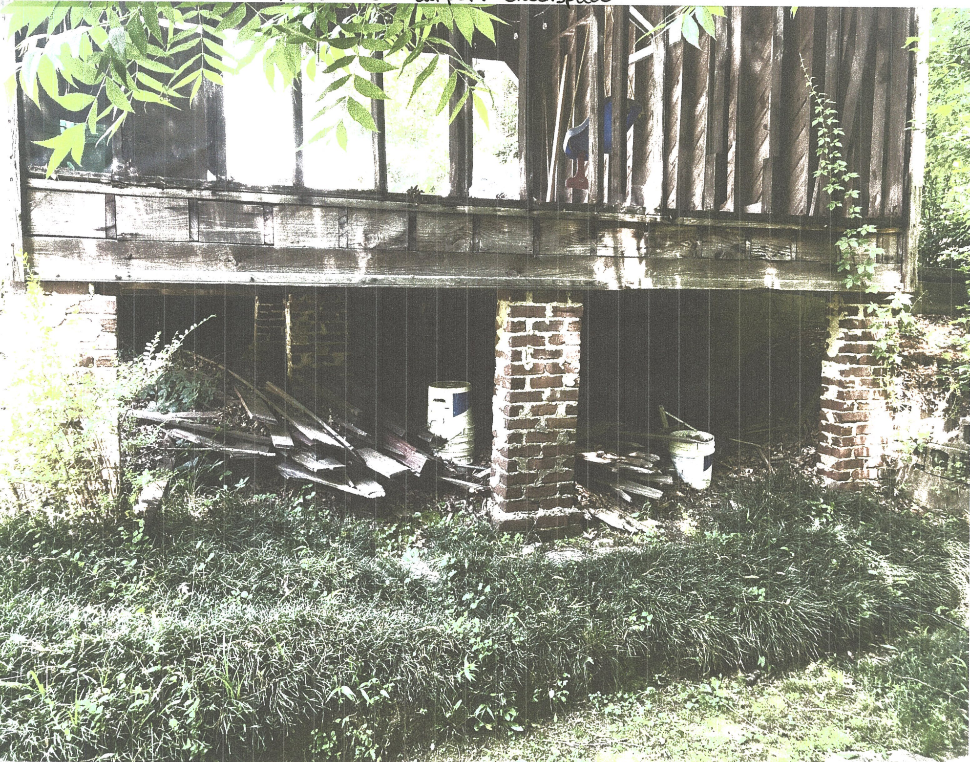
* Picture of carport crawlspace
