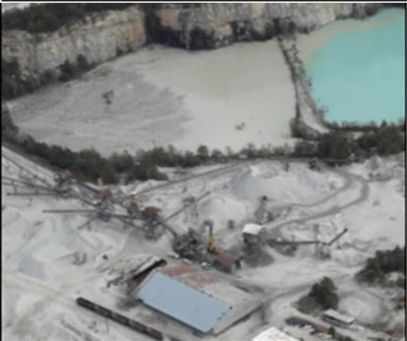
Heavy industrial uses producing noise vibration and dust
