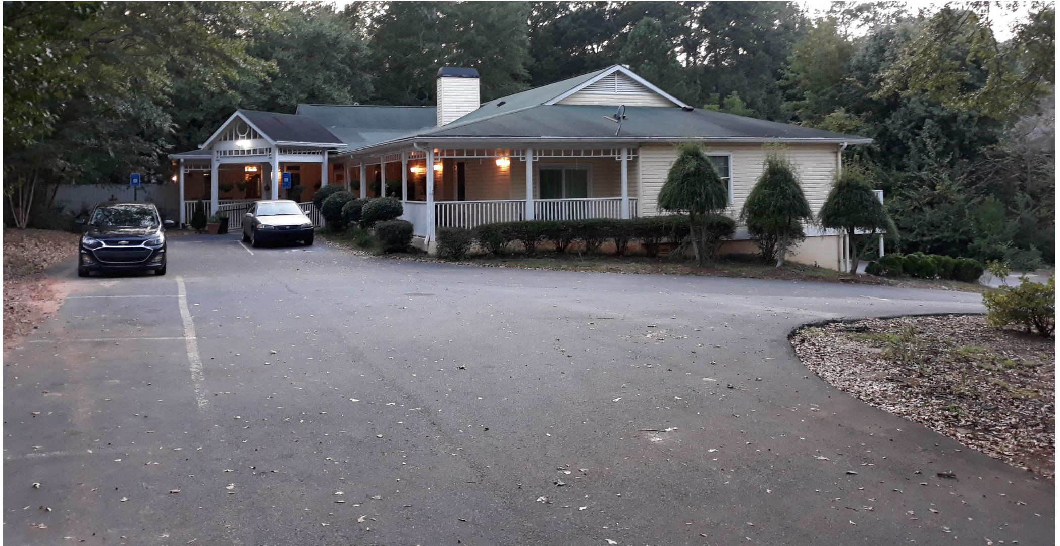
View of Subject Property from Ludovie Lane.
