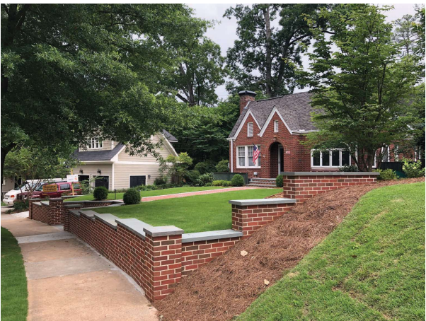
Brick wall with concrete cap
