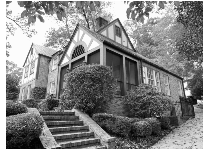
SIDE OF FRONT PORCH - EXISTING
