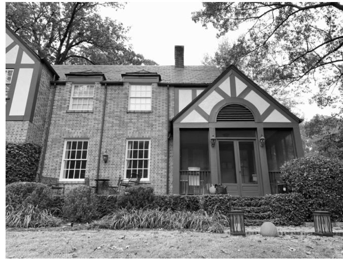
FRONT FACADE - EXISTING
