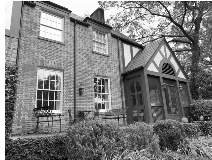
FRONT FACADE & SIDE OF FRONT PORCH - EXISTING
