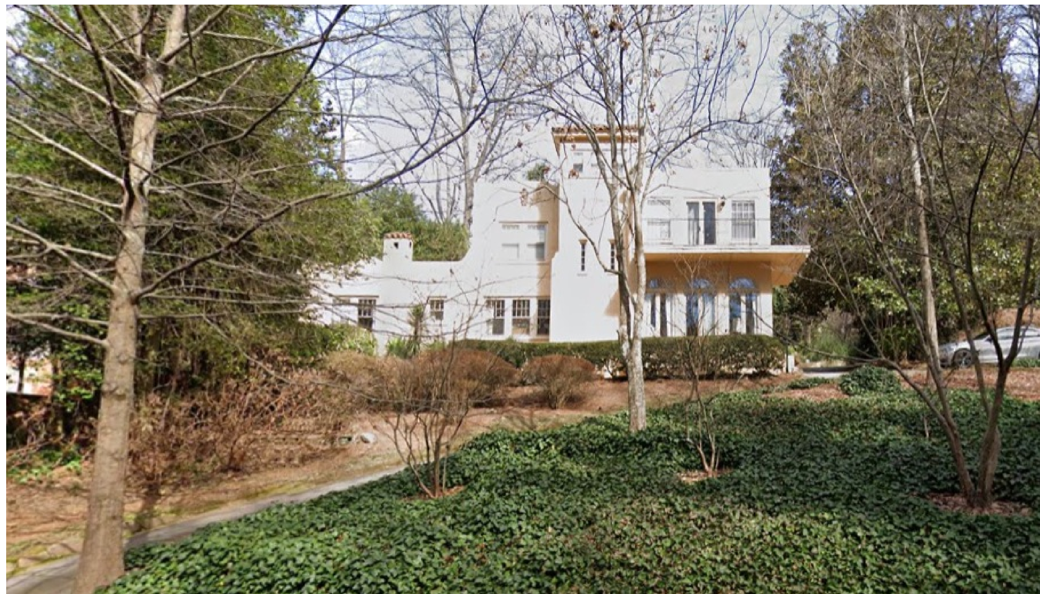
1208 VILLA DRIVE - TO THE RIGHT OF THE SUBJECT PROPERTY
