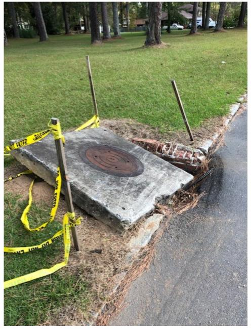
This culvert on Cedar Grove at the end on East Conley was run over by a truck. It has been repaired multiple times but has been in this condition for a few months now.
