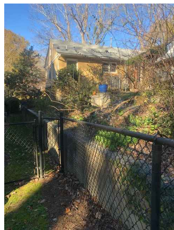
*VIEW TO EAST NEIGHBOR
