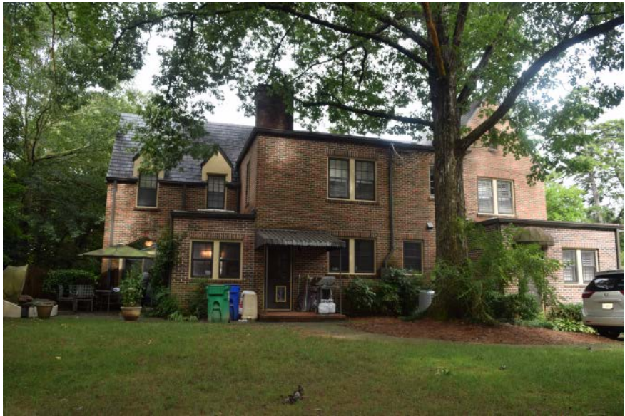
This photo shows the existing rear elevation of the house. The proposed addition goes across this entire rear elevation. This elevation will experience the biggest change in appearance from the proposed work.
