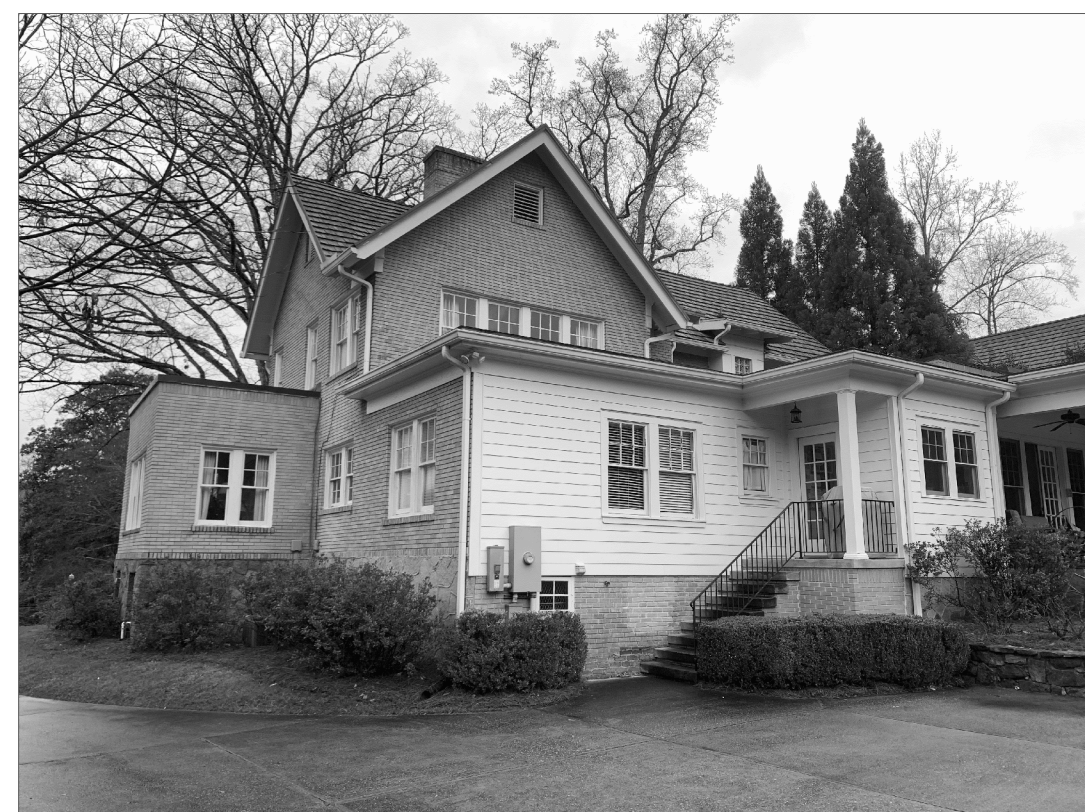
DRIVEWAY SIDE + REAR OF HOUSE
