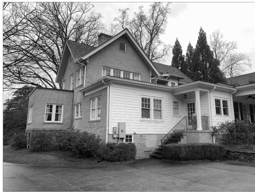
DRIVEWAY SIDE & REAR OF HOUSE
