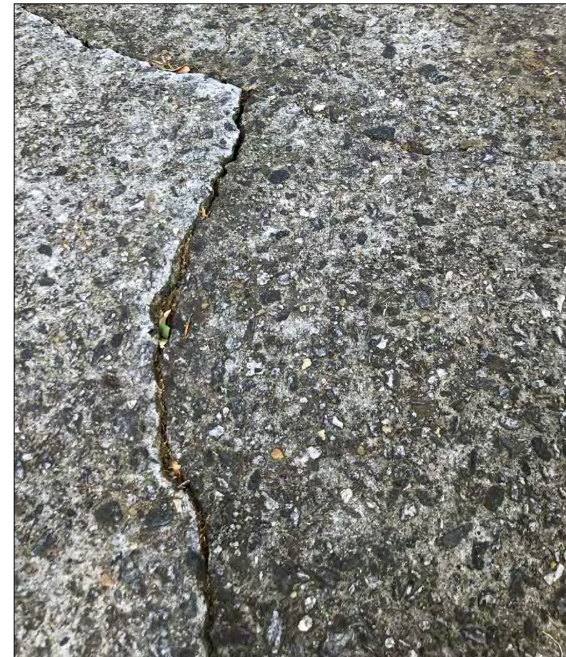
EXISTING DRIVEWAY SHOWING EXPOSED AGGREGATE
