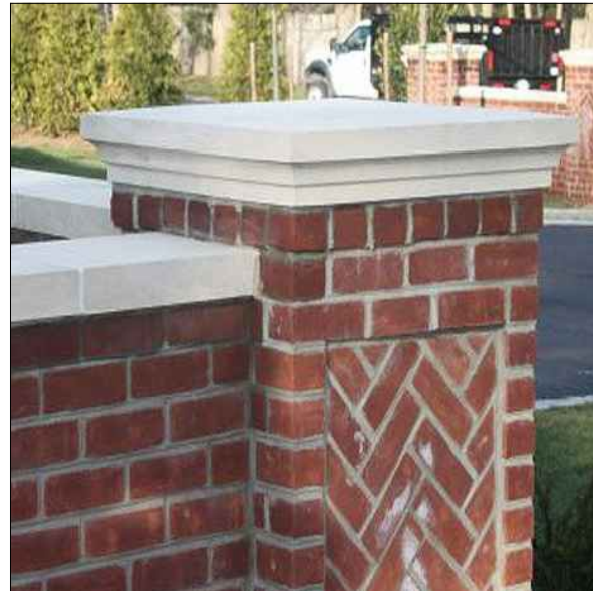
BRICK WALLS + STONE CAP
