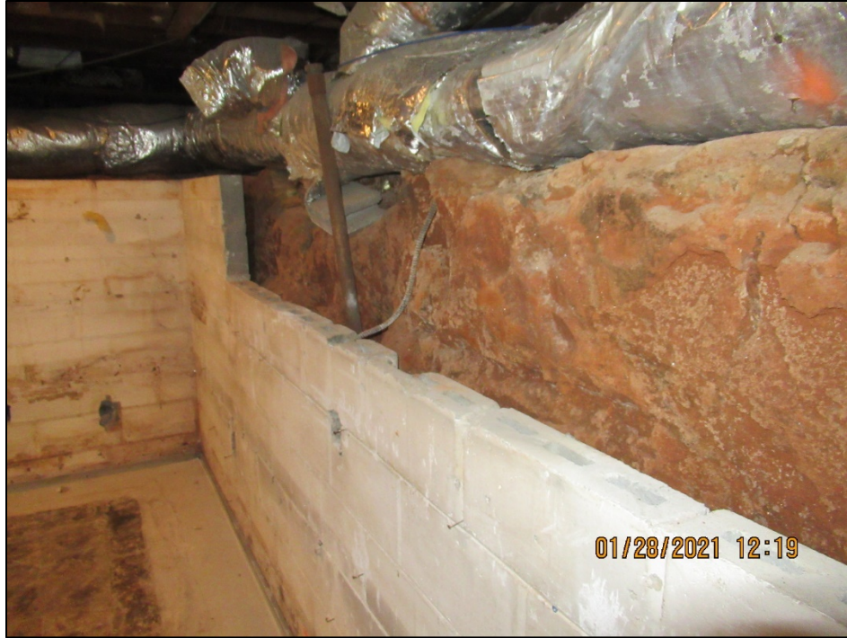
Photo 11: Retaining wall constructed of unreinforced 4" CMU that is close to the exterior foundation walls.
