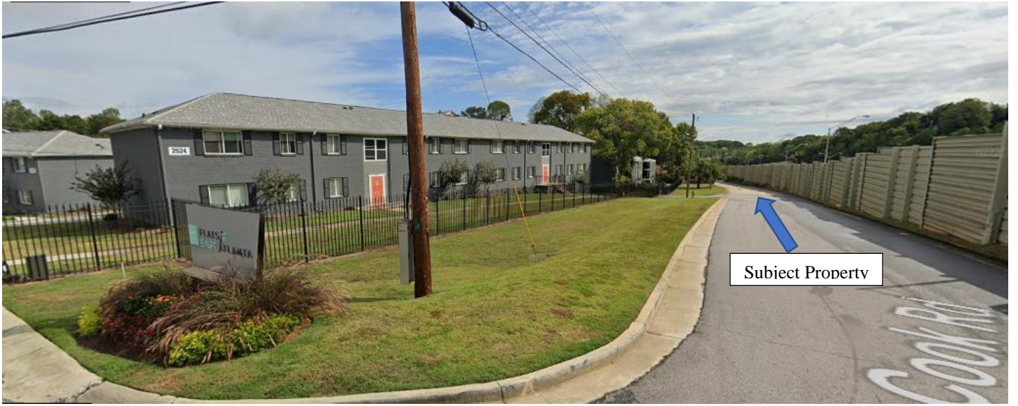
Flats at East Atlanta apartments (on adjoining property to the west)
