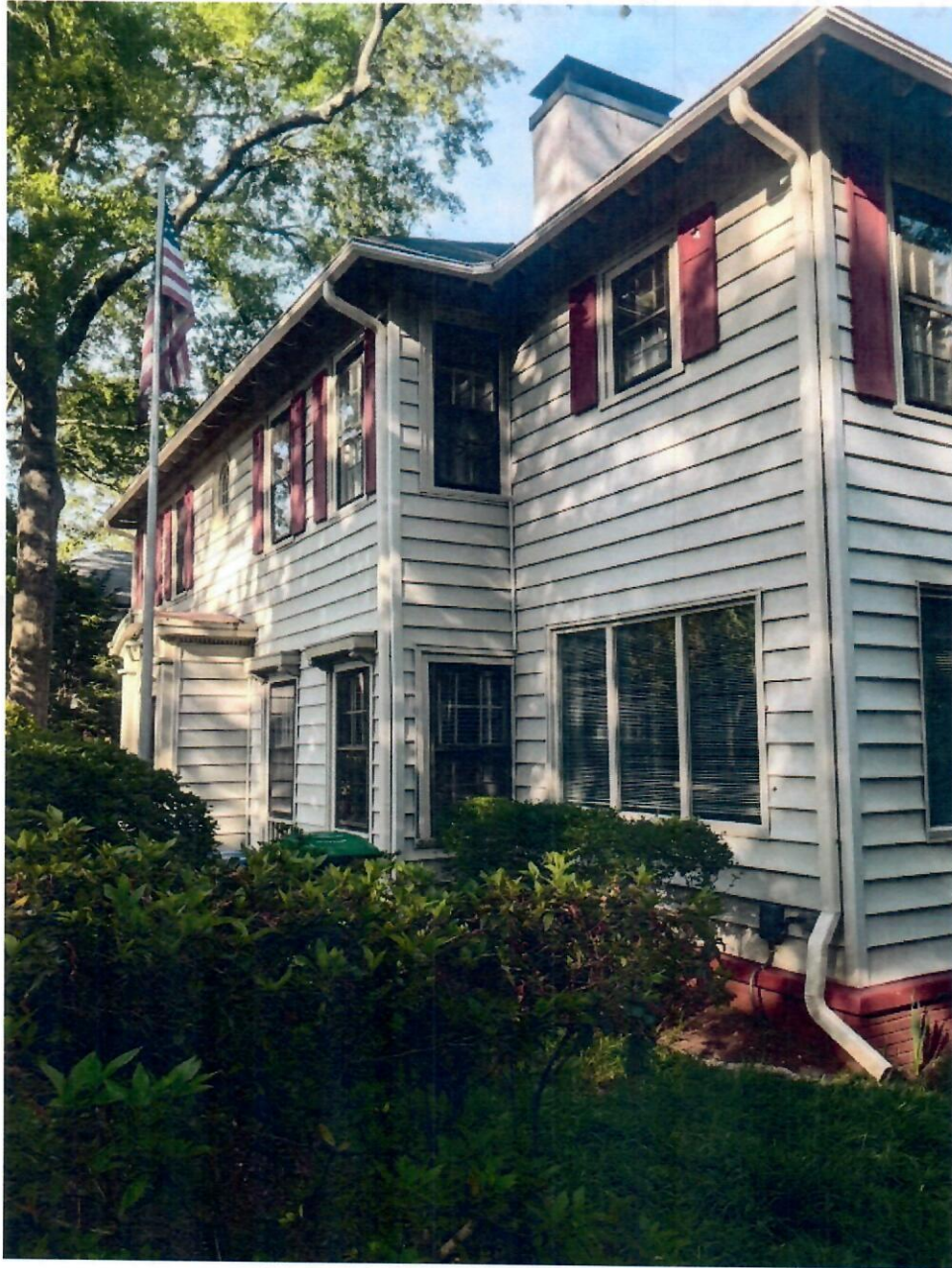
• SOUTH ELEVATION - VIEW FROM DRIVE
