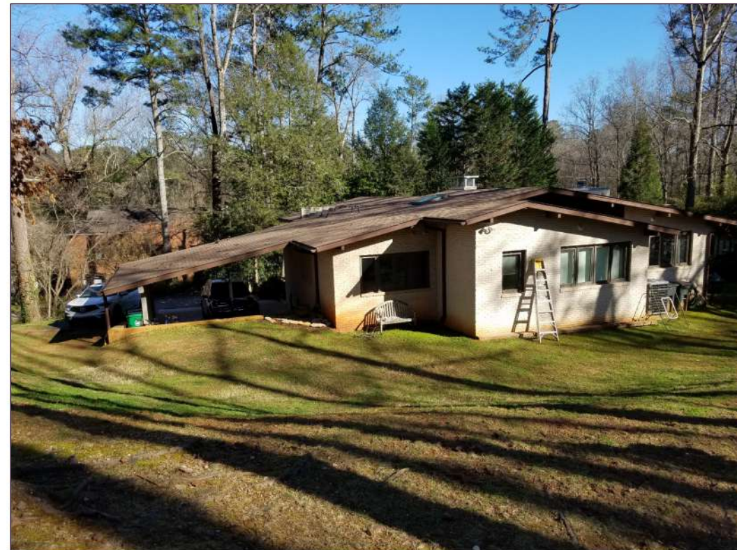
4 WEST FACADE- REAR, FROM TOP OF HILL A 5.02 SCALE: N/A
