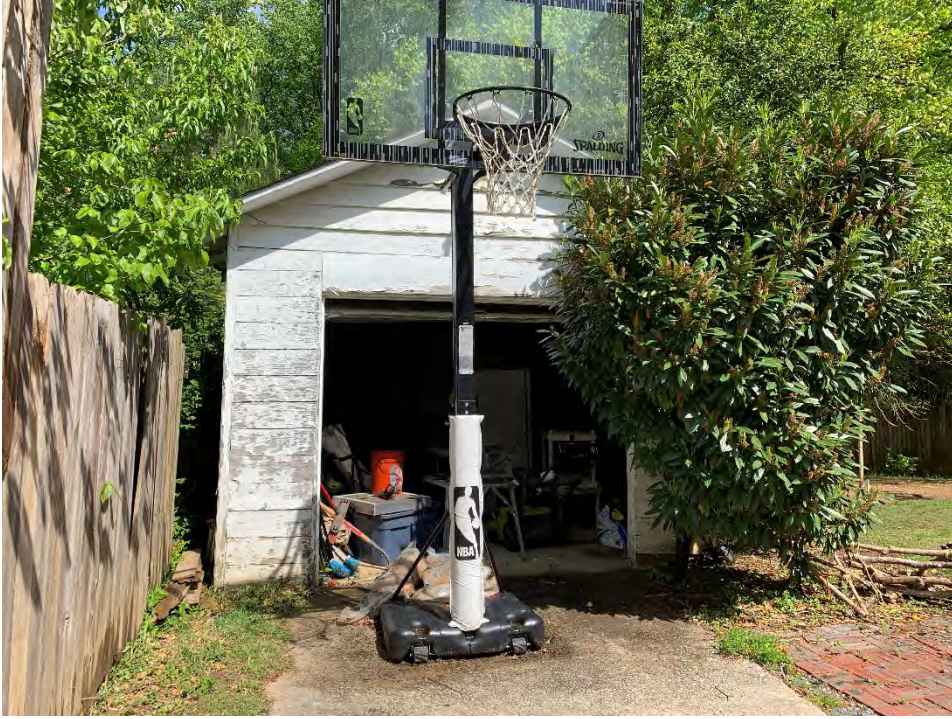
Existing Garage, Front
