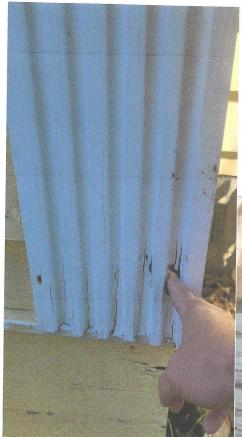
The wood fluted pilasters have extensive termite damage on the 2 corners of the front of the home. One has rotted and broken off and both are beyond repair. No other home in the neighborhood has this faux front. We propose removing the 4 pilasters and placing corner boards. The home would continue to have full length shutters along the front windows.
