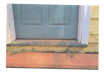
The current front door has been damaged, especially on the bottom. If refinished, the door would be leaky without a seal and inefficient.
