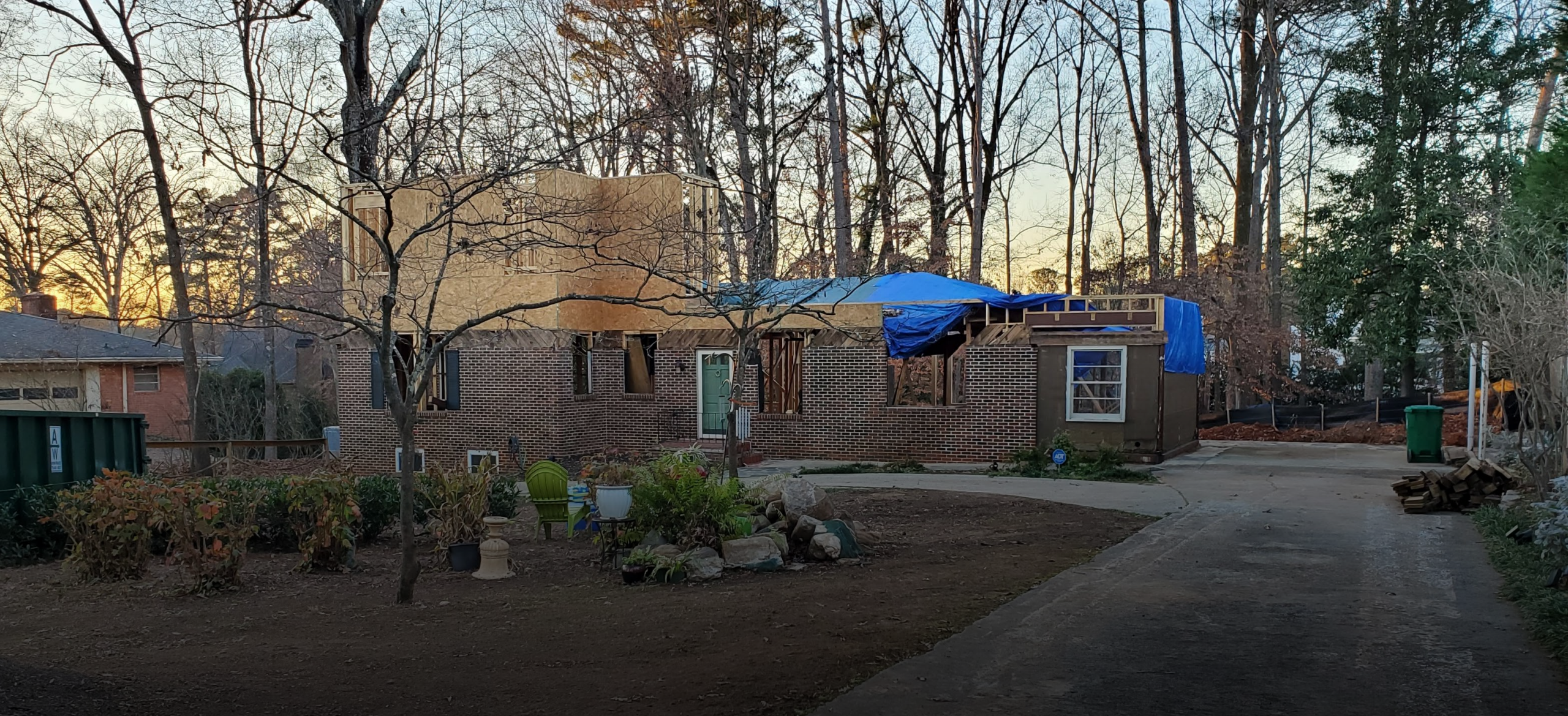
2042 Oak Grove Site Photos
