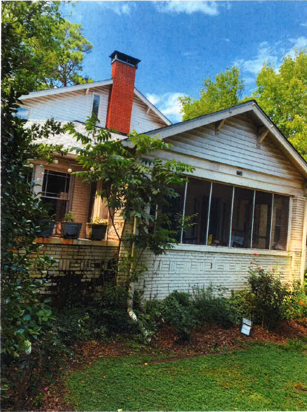
Figure 1: Front view of house from Oxford Road showing vinyl siding at front porch gable, vinyl siding at second floor addition, window at second floor addition, and unpainted brick chimney
