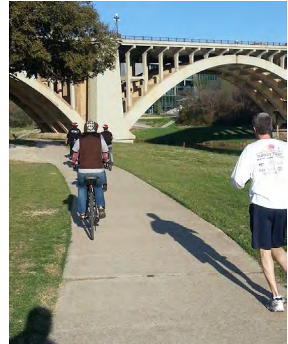
Figure 4mm: Safe Crossings Along Streams and Under Bridges Allow for Additional Pedestrian and Cyclist Connectivity
