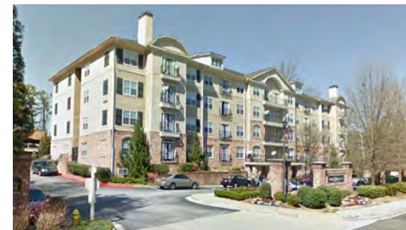
Figure 2j: Multi-family Residential Complex in Study Area
