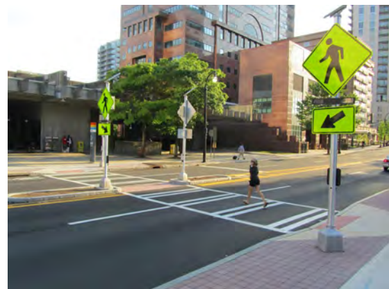
Figure 5c: Midtown Alliance 10th Street RRFB Crossing
