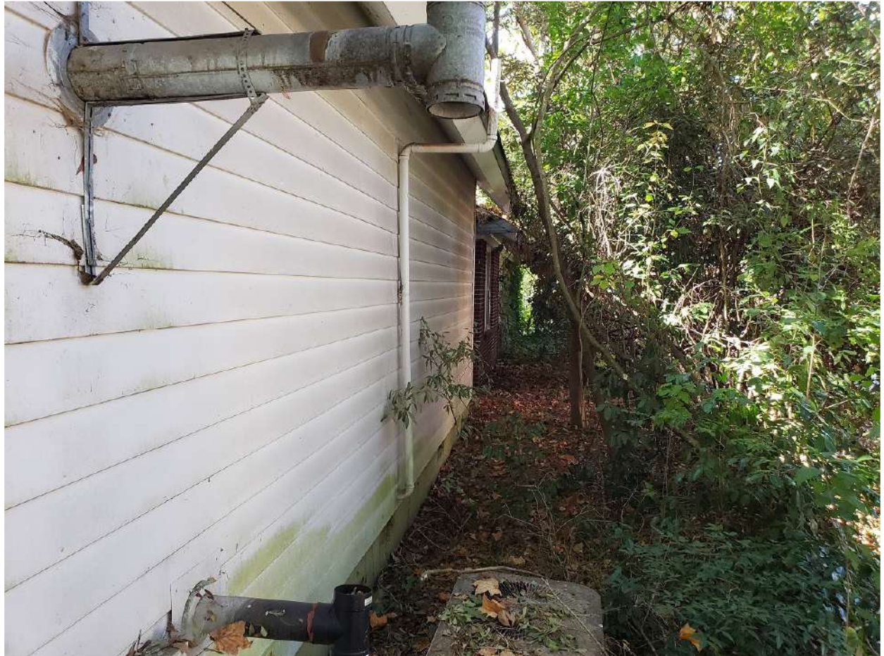
View from rear of northern side – construction of the addition may have prevented drainage from yard
