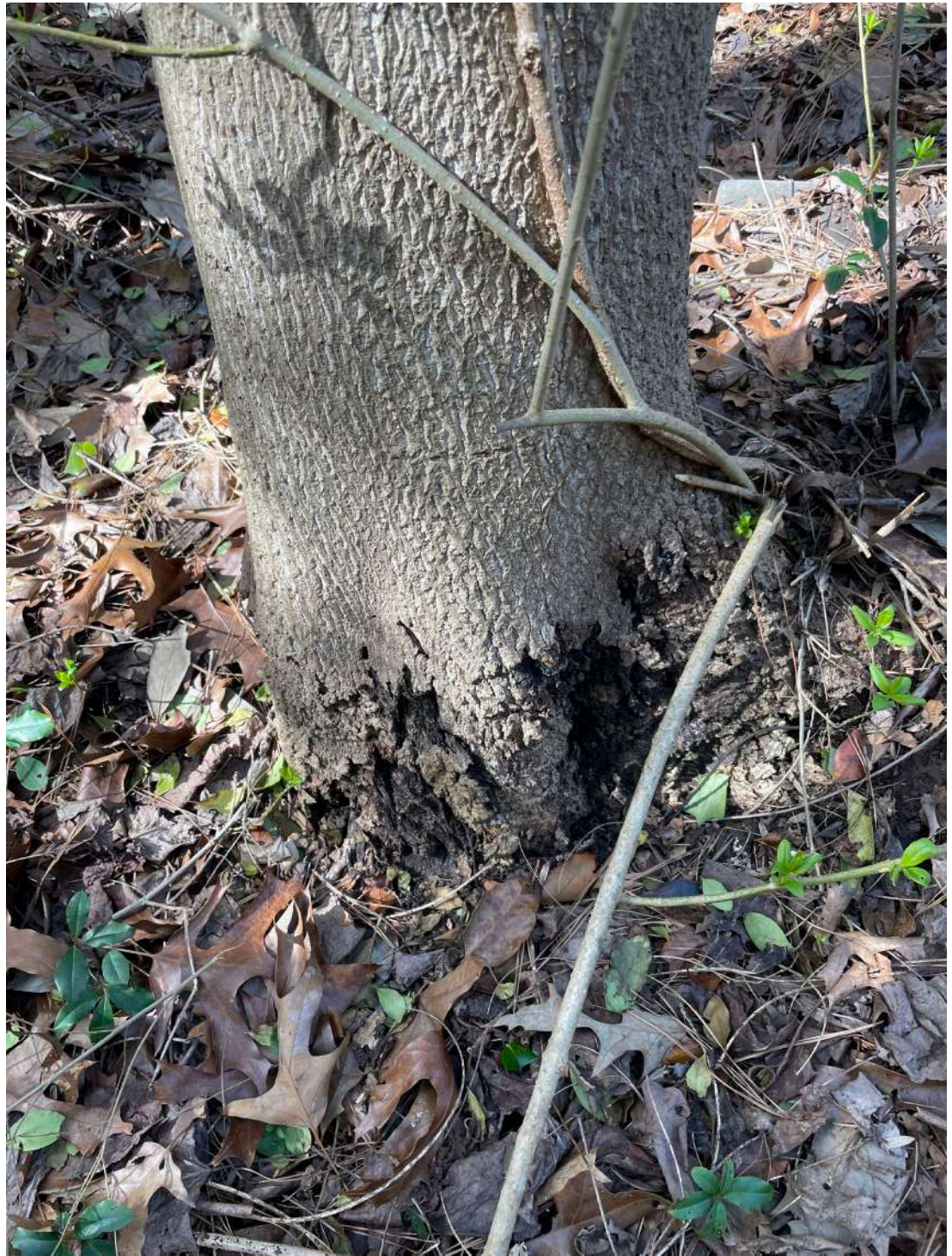
Tree # 29 – Rot and decay present at root crown.
