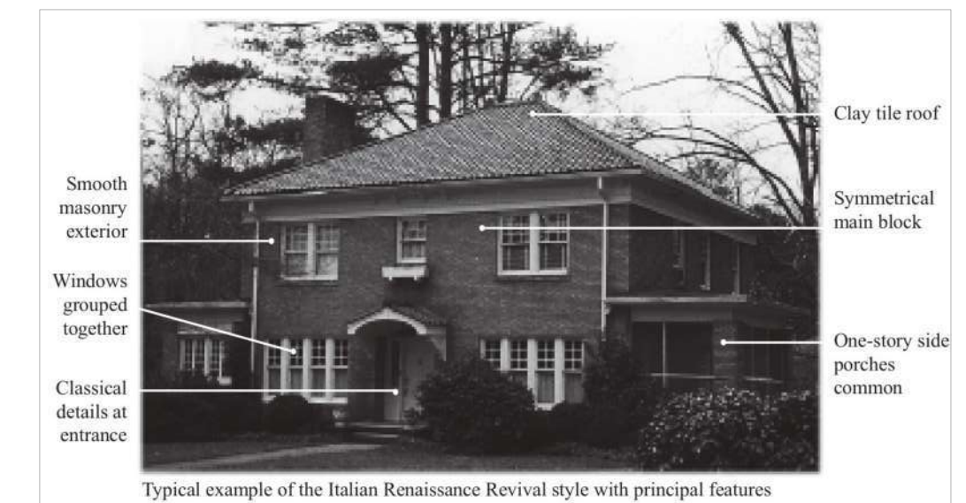
Typical example of the Italian Renaissance Revival style with principal features
