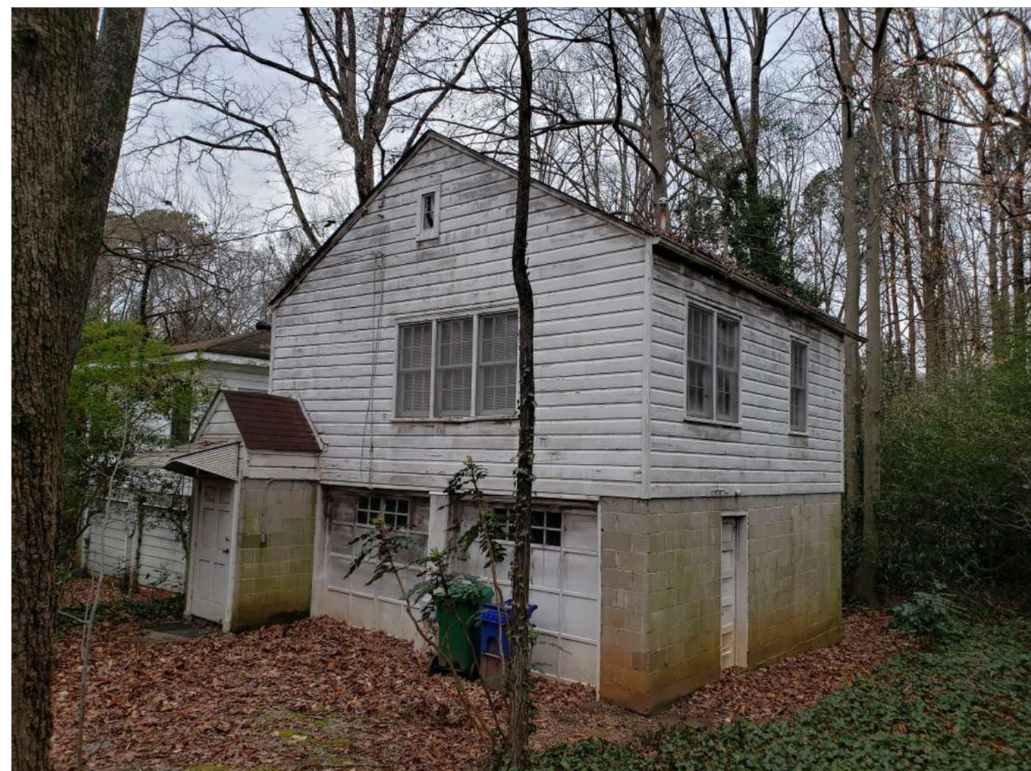
DILAPIDATED GARAGE/ADU. TO BE DEMOLISHED NEW GARAGE / ADU WILL ECHO THIS MASSING (WITHOUT FRONT-FACING GABLE) 186'4" FROM STREET CURB. EXISTING STRUCTURE IS 24' WIDE AND NEW STRUCTURE WILL BE 22' WIDE. THE LOT COVERAGE OF THE NEW ACCESSORY STRUCTURE AND NEW DRIVEWAY WILL BE LOWER THAN EXISTING ACCESSORY AND DRIVEWAY.
