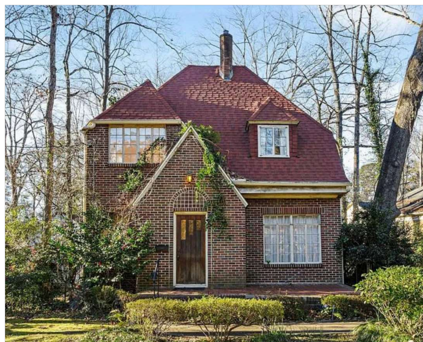
NEIGHBORING TWO-STORY HOUSE - APPROX. 28' WIDE THE NEIGHBORING HOUSE HAS A VERY TALL RIDGE ON ITS HIP ROOF AND THE FLOOR IS 5' ABOVE OUR PROPOSED MAIN FLOOR ELEVATION, DUE TO OVERALL TOPOGRAPHY
