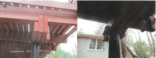
The outer girder/ beam serving the deck lack protection against movement/ deflection and proper attachment between the support post and deck members. Rusting and damage was noted at the top of the supports.
