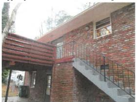
Excessive openings were noted in railings at the deck area with low railing height present in areas and loose railings present.
