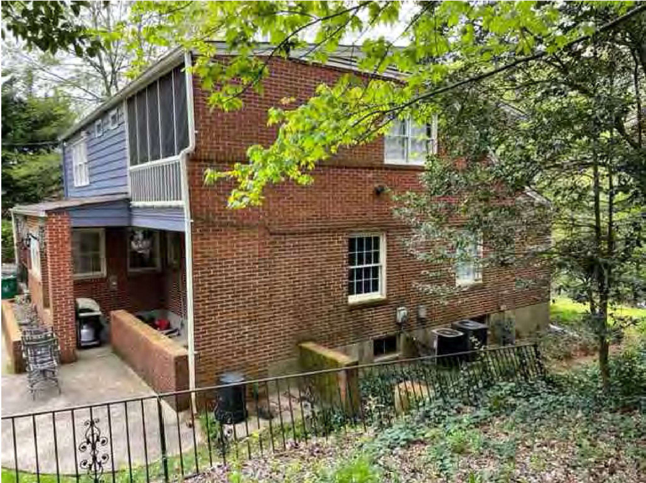
WEST SIDE OF HOUSE FACADE
