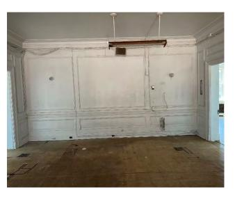
IMG 209-2: Applied Panel molding on plaster over raised panel wainscot in Stair Hall runs throughout second floor circulation hallways.
