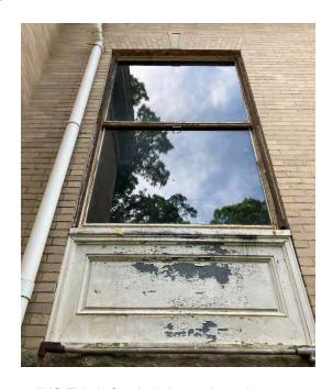
IMG EX5-2: Steel window and panel insertion in the Banquet Hall showcasing the material specificity in the addition on the mansion's north side.
