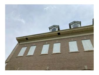
IMG EX3-4: Jack arch windows in the children's rooms above the Solarium. Brick on Southeast side is largely in good condition.
