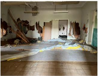
IMG 311-4: Current condition of one of the subdivided rooms in the middle of the ballroom. Note ACT flooring over original wood flooring to be removed. Wood floors may be restorable if plywood subfloor was utilized under tile but assume carpet finish for SD pricing.
