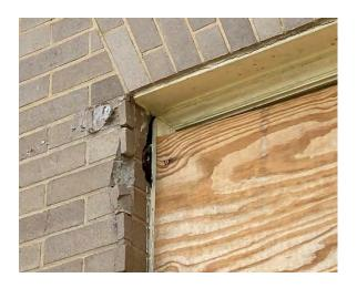
IMG EX6-3: Crumbling wood on the top corner of a jack arched window.
