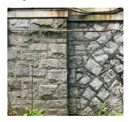
IMG EX5-3: Stone base moving from logical to random pattern on the north side.
