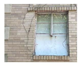
IMG EX6-5: Broken steel window on the Organ Room; typical for many steel and wood windows around the property.
