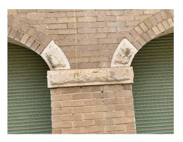
IMG CH2-3: Garage door trim connection with brick arch leading into stone base.
