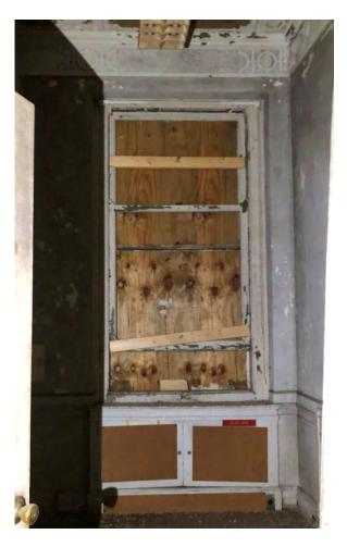
IMG 111-2: The space is currently divided up into various office spaces used in the institution era. This wood window will be removed to create an opening to a new LULA elevator in Lightwell 1.
