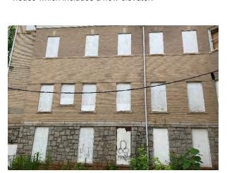
IMG EX2-3: Boarded up windows cover the East Wing of the Candler Mansion, largely protecting the broken windows that lie behind.
