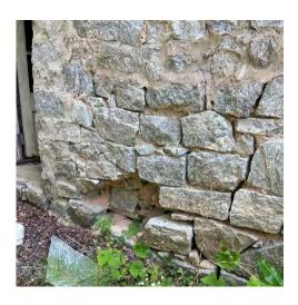
IMG CH3-1: Missing and cracked stone on basement level.
