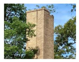
IMG CH3-3: Replacement needed on chimney with bricks missing on the top.
