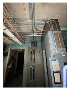
Figure 4: Branch circuit panelboards on Basement Level
