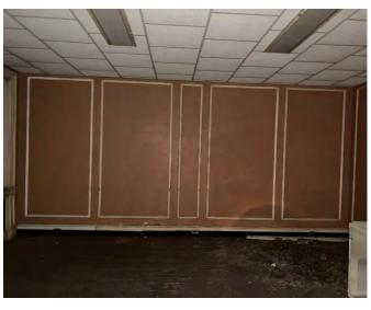
IMG 203-2: Paneling on the walls and crown molding hidden by institutional installation of ACT ceilings in all second-floor rooms and wing corridors.
