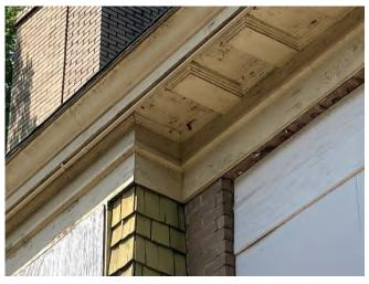
IMG CH2-4: Corner where deteriorating paneling connects with trim as well as brick wall.
