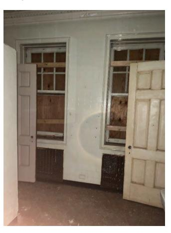
IMG 204-2: Recessed radiator enclosures with cast iron grilles below windows. Ornamental tile casing at windows and doors. Ornamental tile crown mouldings. (all with epoxy coatings to be removed)
