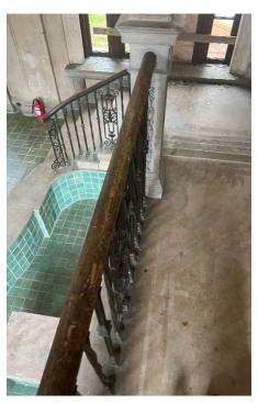
IMG 101-2: Concrete stairs and original railing leading down into Solarium. Fountain element integrated into stair design.
