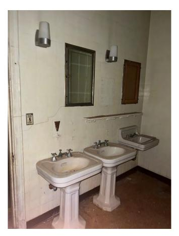
IMG 204-1: Typical bathroom with epoxy coated original tile walls and Traffic Coating on original tile floors covering specific bathroom floor tiles.
