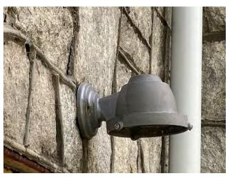
IMG CH2-2: Close up of stone on Carriage House with fixture and pipe running along. Original fixtures are going to be maintained in restoration.
