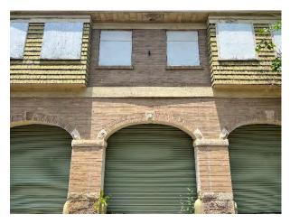
IMG CH1-1: East facing, front portion of Carriage House. Deteriorating roof trim and paneling need to be fixed.
