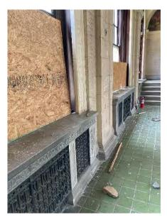
IMG 101-4: Rusticated stone veneer pilasters and typical arched opening carved detailing.
