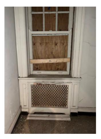
IMG 206-1: South Hallway with typical radiator enclosure as seen in most of the mansion. (this window was originally in end bedroom on this wing but became part of egress corridor when stair was added to end of wing.)
