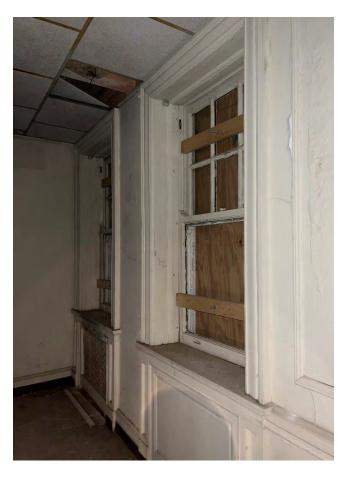
IMG 206-2: South Hallway paneled wainscot and wall panel molding. Glazing "removed" at majority of windows to install exterior plywood security coverings.
