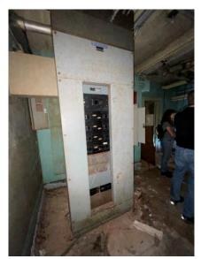
Figure 3: Existing Building Main Switchboard
