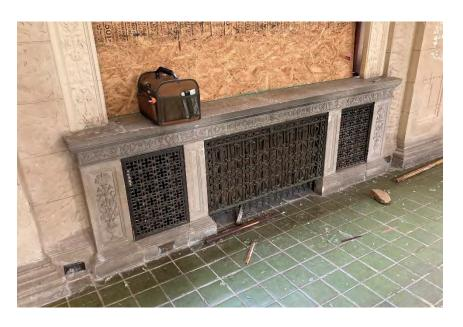
IMG 101-3: Cast stone radiator enclosures with cast iron grilles.
