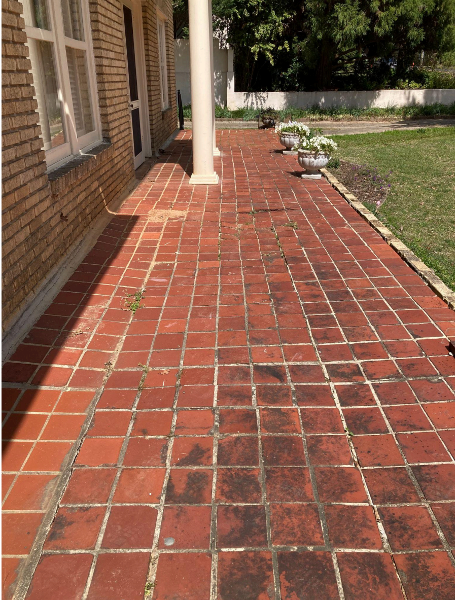
Existing conditions: View of tile porch/terrace from the south
