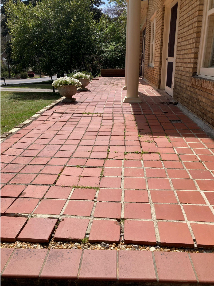
Existing conditions: View of tile porch/terrace from the driveway
