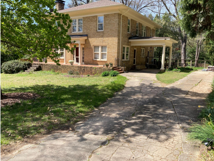
Existing conditions: view from street of 1228 Oxford Rd NE
