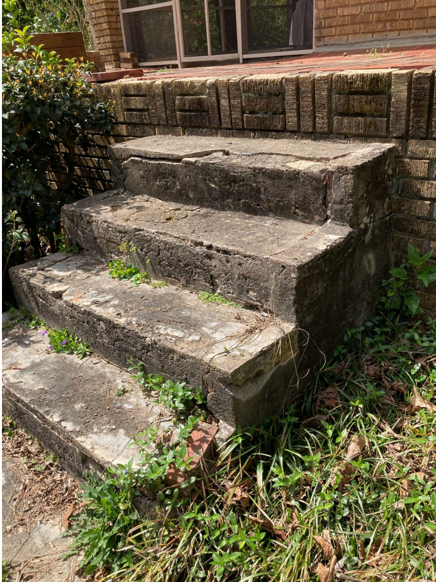
Existing conditions: Non-historic concrete stairs to be removed
