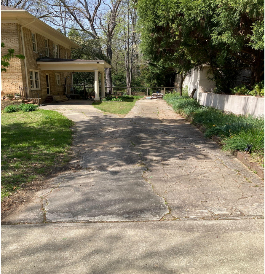
Existing conditions: driveway
