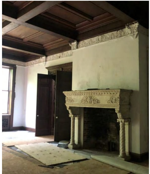
IMG 122-2: Opening to Music Hall (remove non-historic doors) Carved marble fireplace to be cleaned and restored.
