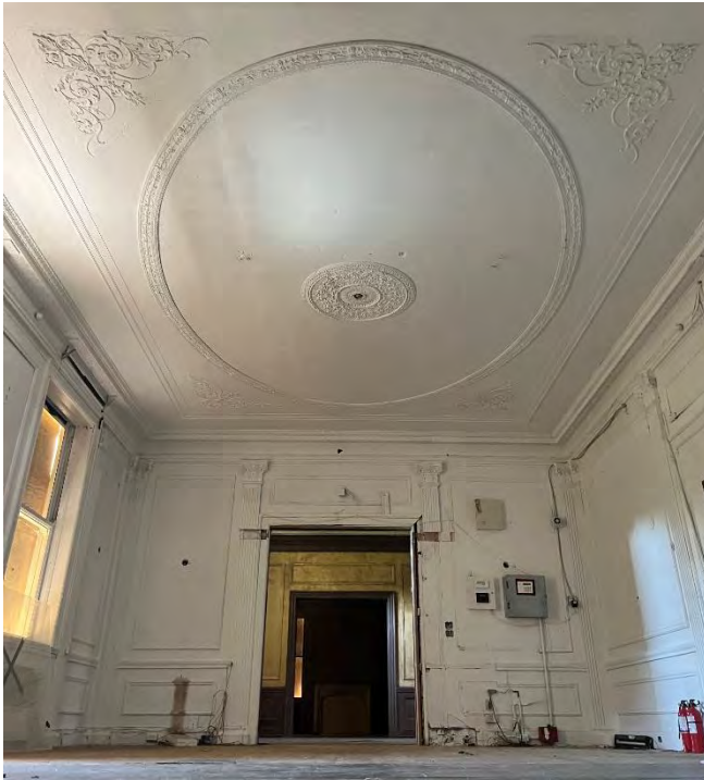
IMG 110-1: Formal Dining Rm- Intact plaster molding.
