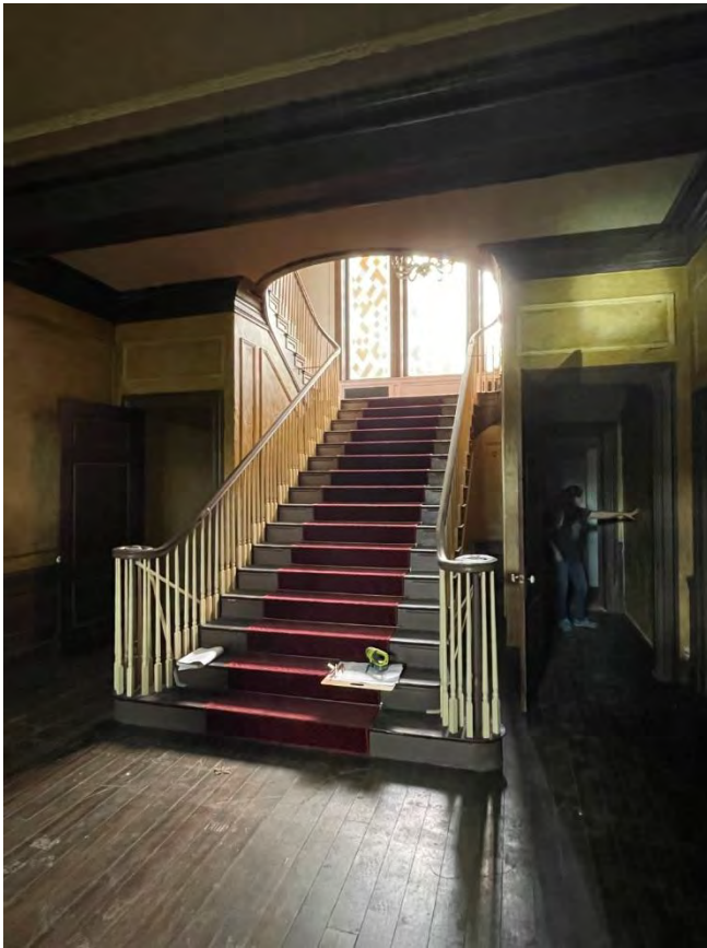
IMG 109-1: Entry Hall Main Stairs. Remove Non-Historic infill under 2 nd stair runs. Remove/replace non-historic rail and balusters. Visible flooring is loose laid LVT plank over original 1 1/2" T&G wood flooring.
