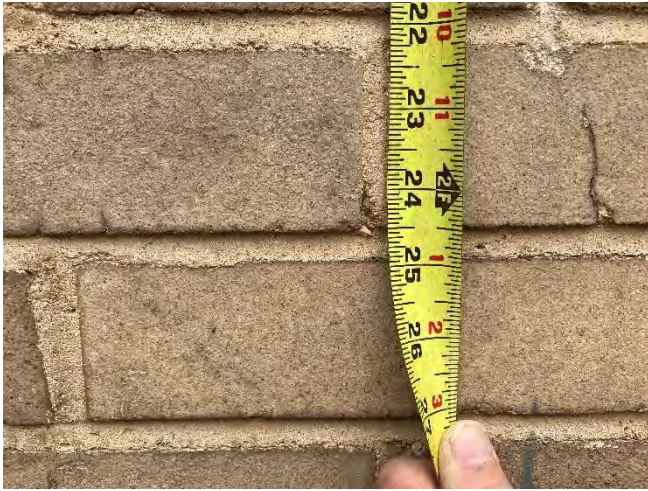
IMG CH2-1: Typical size of brick in both the Main House and Carriage House.
