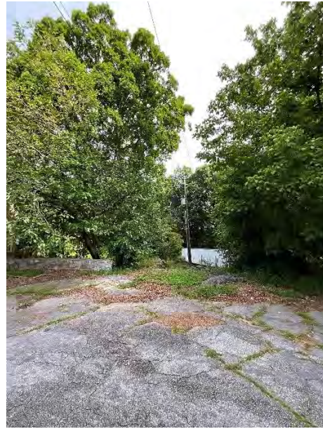
Figure 2: Existing Single-Phase Overhead Electrical Service – Back Buildings
