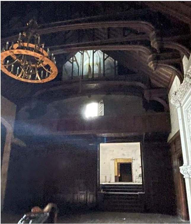
IMG 120-1: Music Hall looking south towards Main House. Wood paneled walls and vaulted ceiling, balcony.
