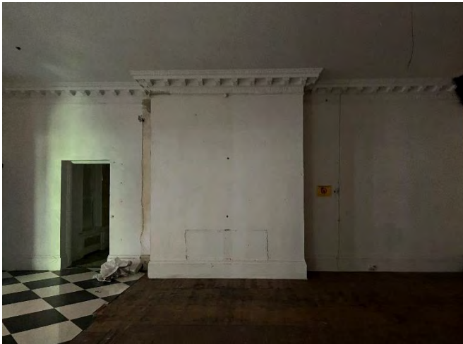
IMG 102-3: Previous fireplace location.
