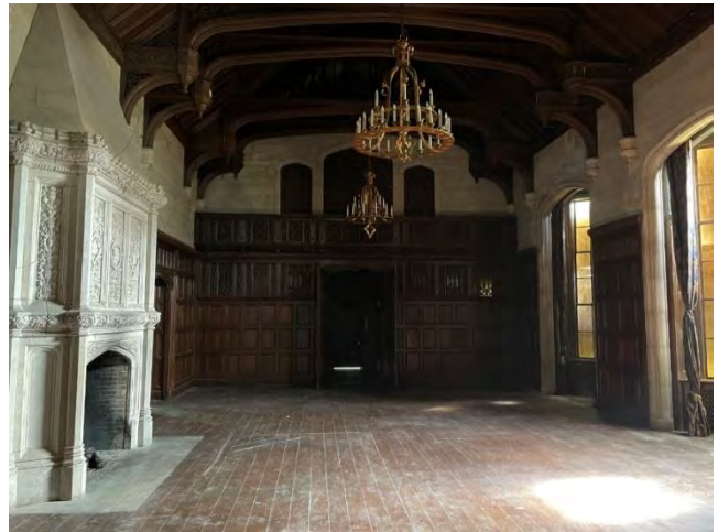
IMG 120-2: Music Hall looking north towards original Organ Room. 6" ornamental wood plank flooring, stone arched openings to tall bay windows front of mansion.
