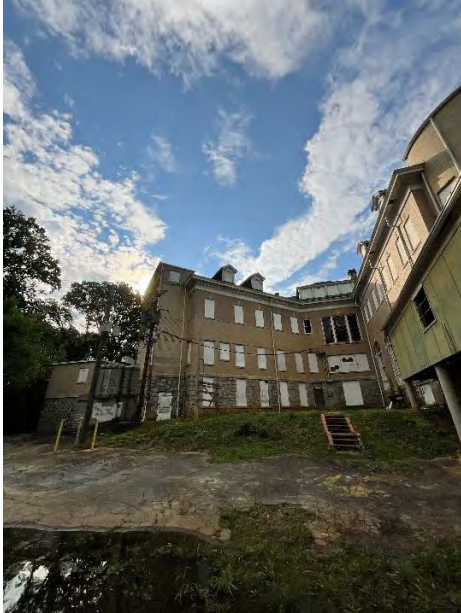
Figure 1: Existing Overhead Electrical Service - Main Building
