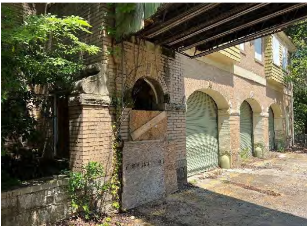
IMG CH1-3: Connection point between bridge from Solarium to second floor. Previous entry below now boarded up.
