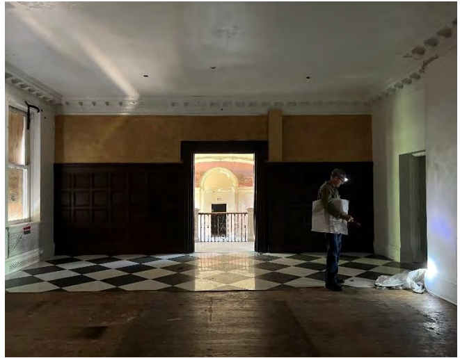
IMG 102-2: Family Living Room looking west towards Solarium. Black and white tile, paneling, and textured paint are non-historic movie set additions.
