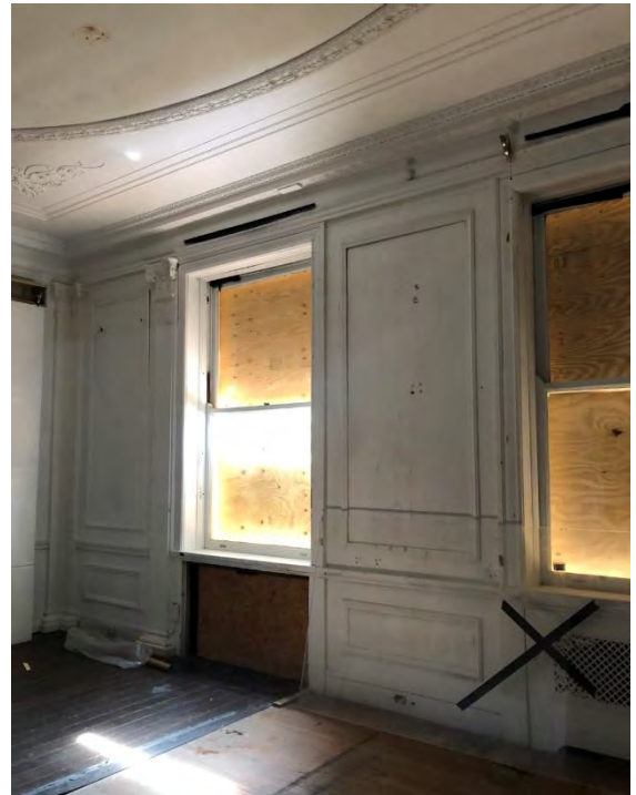
IMG 110-2: Paneling on walls- Formal Dining Rm.
