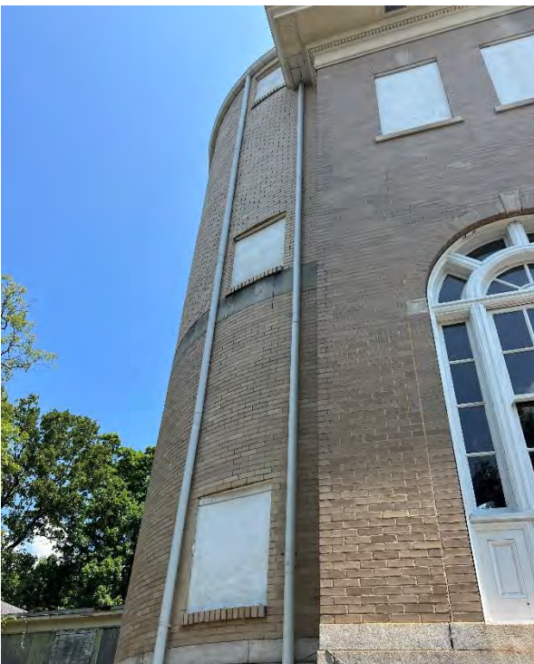
IMG EX3-3: South Stair addition onto Solarium.
