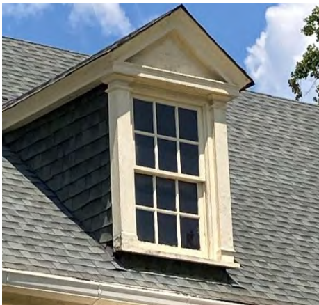
IMG EX5-4: Dormer type above the music hall. Other dormers on the third floor are similar but with arched trim.
