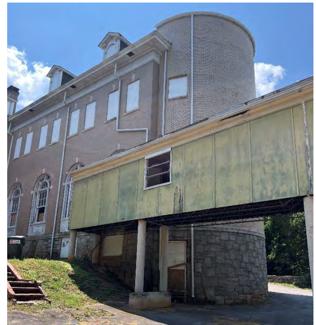
IMG EX2-4: Closer look at the Solarium half circle stair addition as well as the addition of the bridge that connects to the Carriage House.
