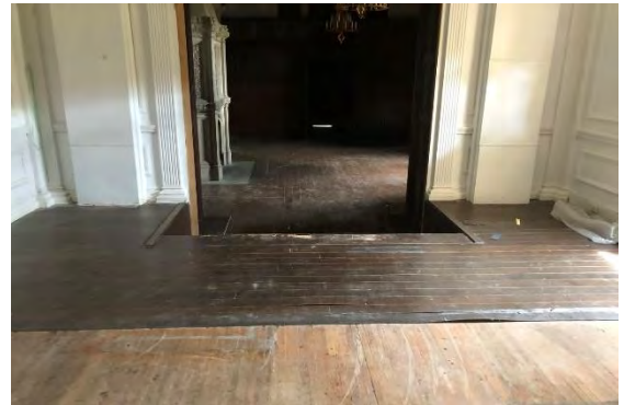
IMG 110-4: Stairs over Original to be removed.
