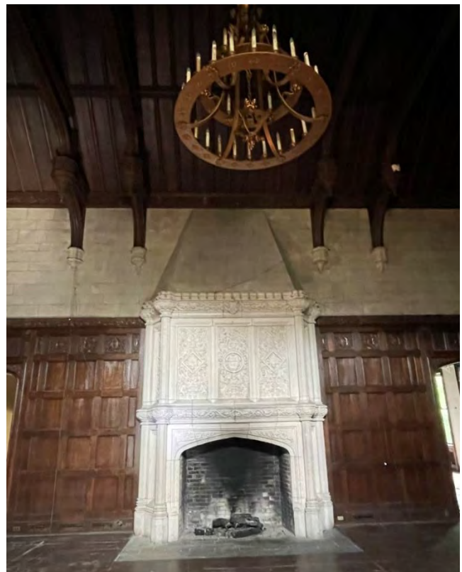
IMG 120-4: Stone Fireplace and stone veneer walls above paneling.
