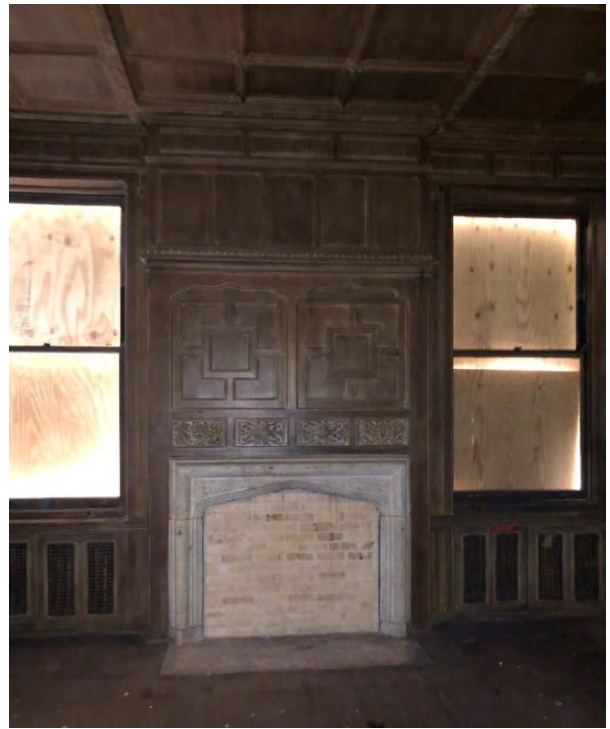
IMG 104-2: Filled in fireplace with paneled radiator covers below windows.
