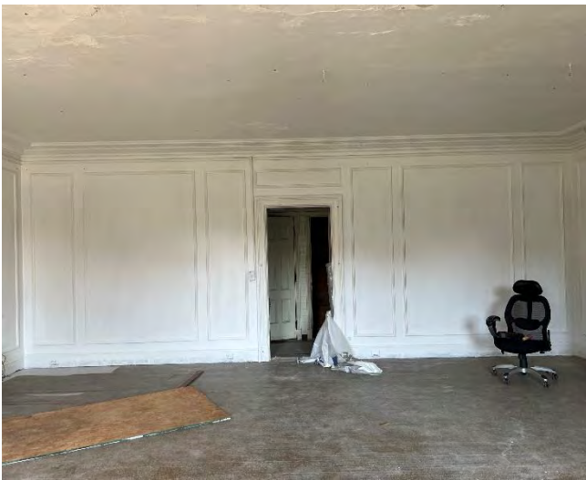
IMG 208-3: Majority of the second floor T&G wood flooring and bathroom tile is covered in a heavy-duty fluid applied traffic coating.
