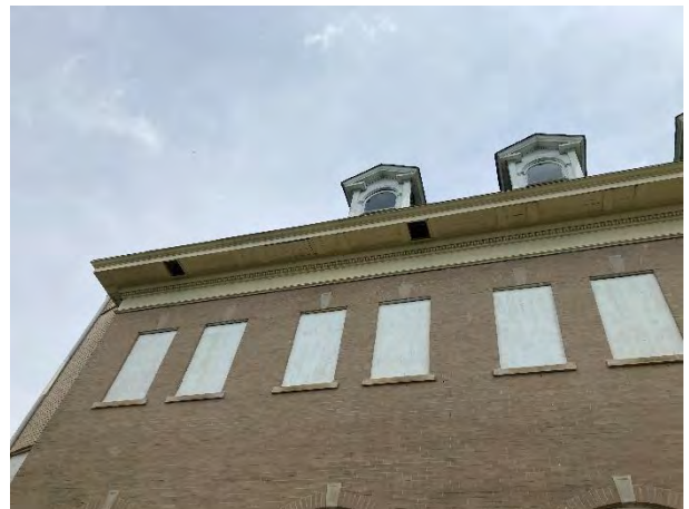
IMG EX3-4: Jack arch windows in the children's rooms above the Solarium. Brick on Southeast side is largely in good condition.
