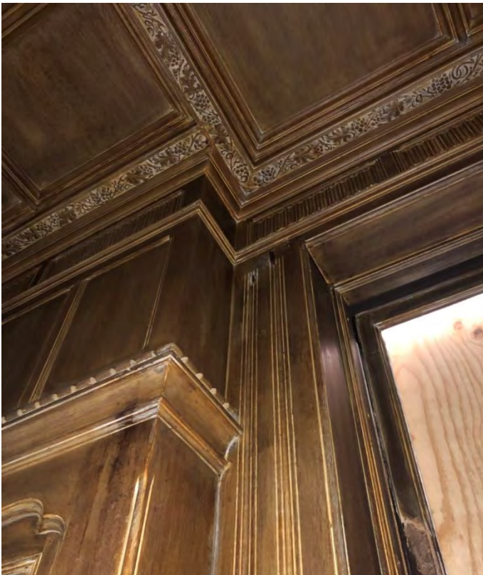
IMG 104-3: Heavily detailed trim in good condition.
