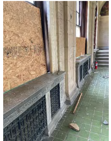
IMG 101-4: Rusticated stone veneer pilasters and typical arched opening carved detailing.
