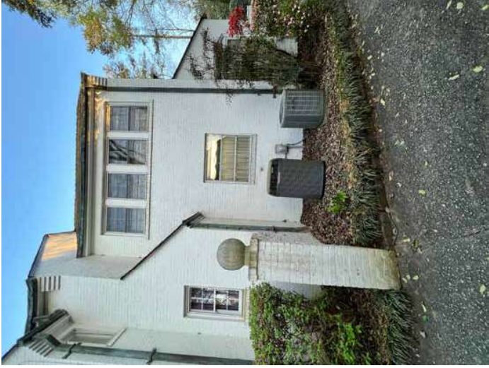
EXISTING MUD ROOM @ SIDE TO BE REMOVED AND RENOVATED
