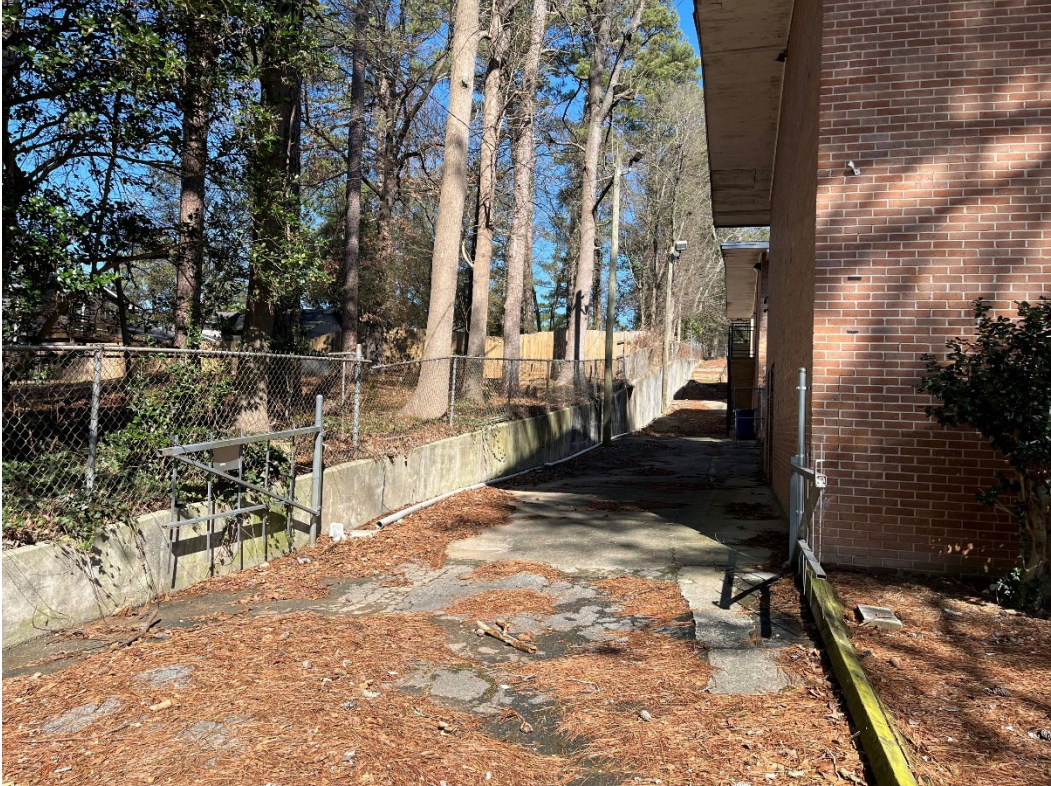
Existing west side elevation, as seen from the driveway at the back of the buildings:
