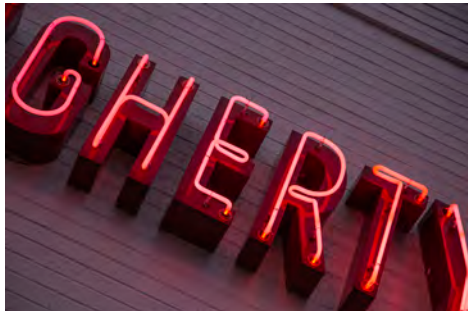
OPTION 7A: Exposed Neon Mounted Directly to Façade OPTION 7B: Exposed Neon Mounted on Solid Letter Forms
