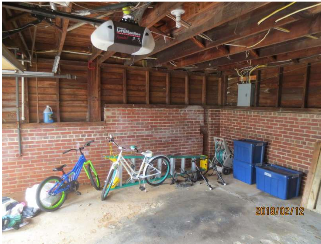
Left foundation wall and over-spanned 2x12 joists
