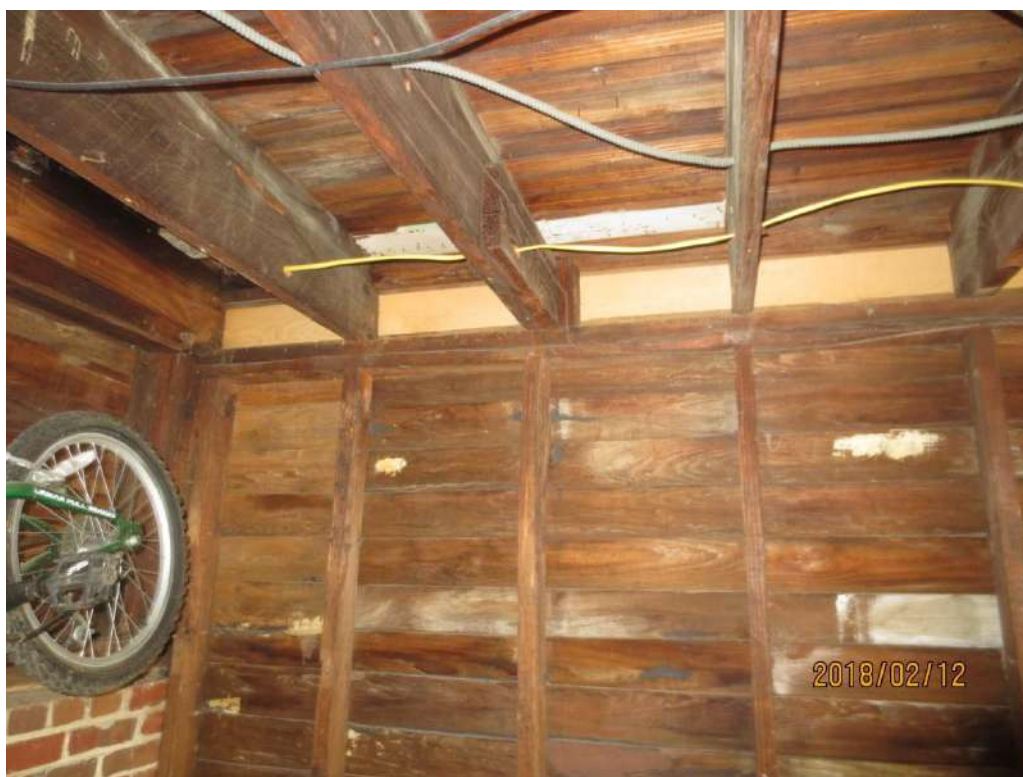
Damaged wall framing to be replaced
