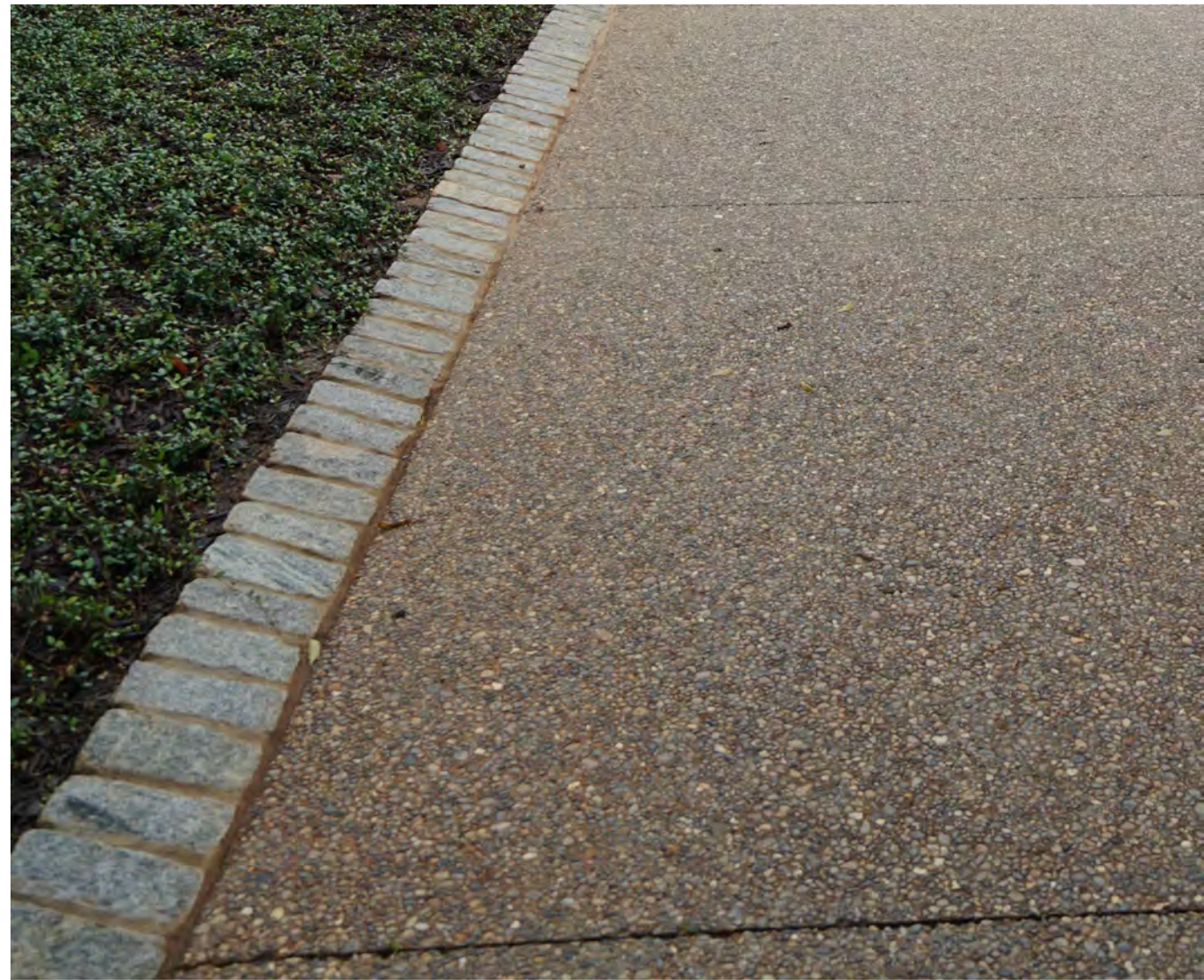
EXPOSED AGGREGATE MOTORCOURT WITH COBBLESTONE BORDER
