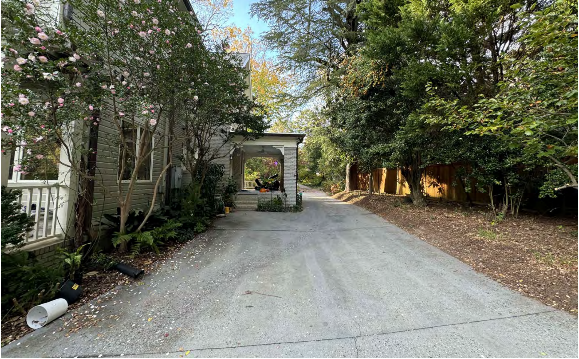
NORTH SIDE OF MAIN HOUSE FACING STREET
