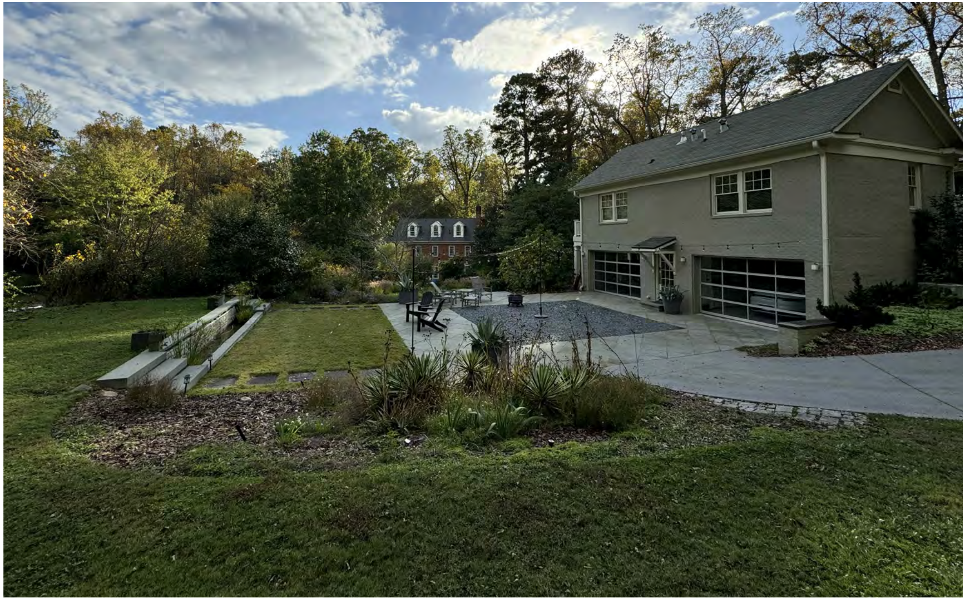
SIDE & REAR OF EXISTING GARAGE / GUEST HOUSE
