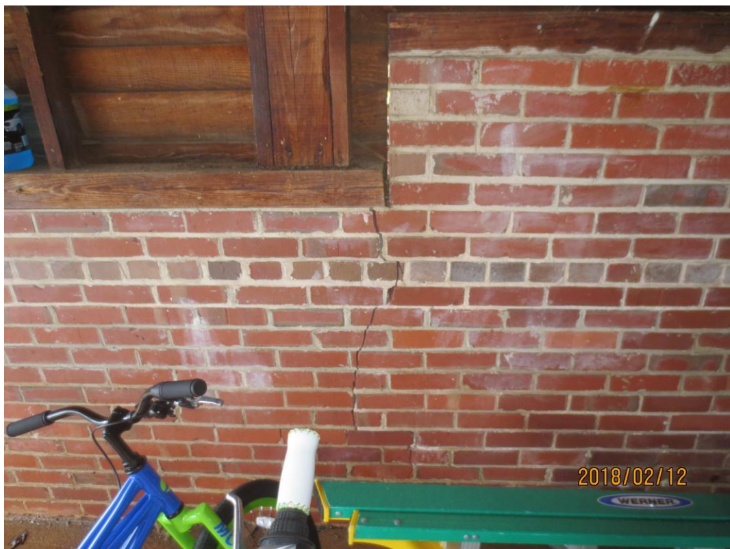
Left wall settlement crack, new underpinning footings required.
