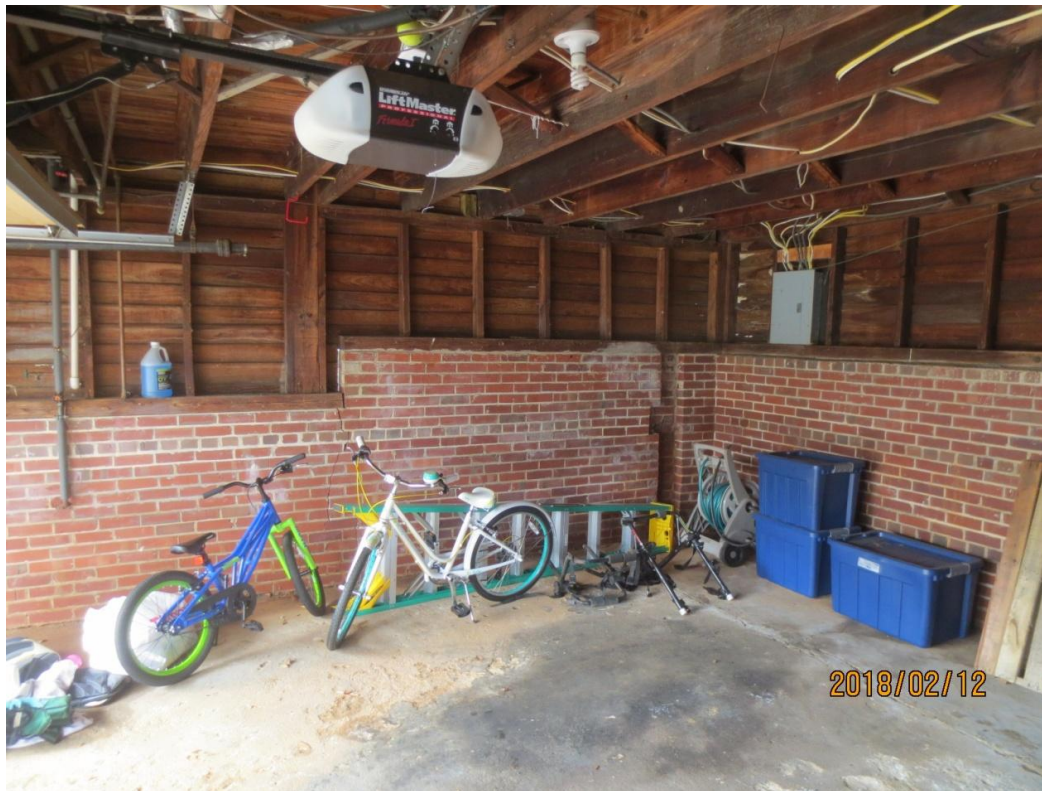
Left foundation wall and over-spanned 2x12 joists
