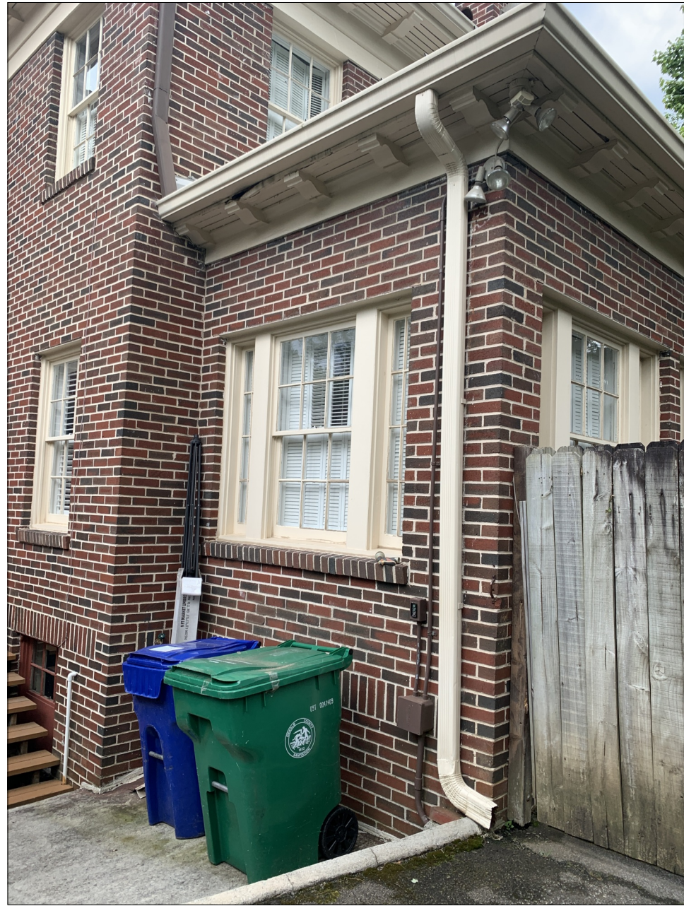
CONCRETE LANDING SLOPES TOWARDS BASEMENT WINDOW
