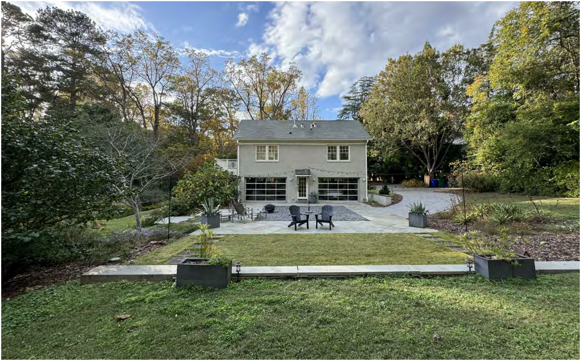
REAR FACADE OF EXISTING GARAGE / GUEST HOUSE
