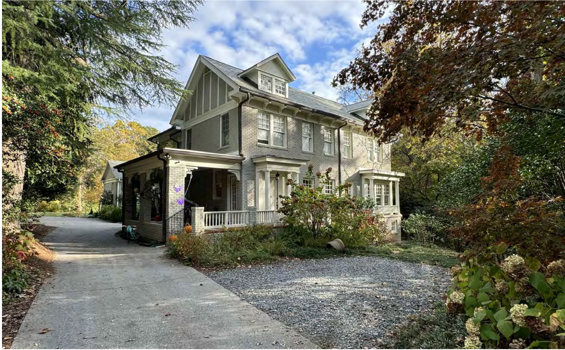
FRONT FACADE OF MAIN RESIDENCE
