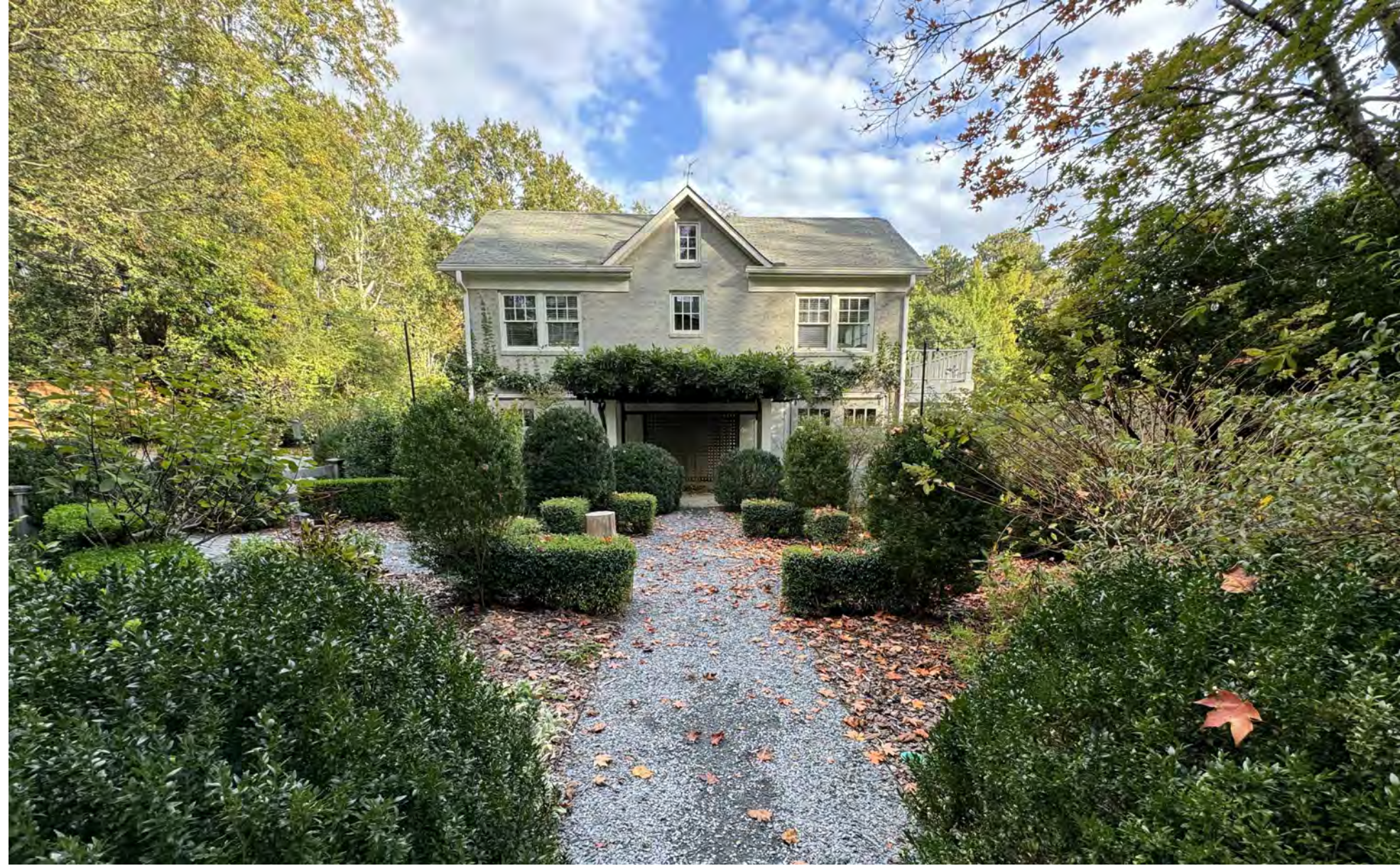
FRONT FACADE OF EXISTING GARAGE / GUEST HOUSE
