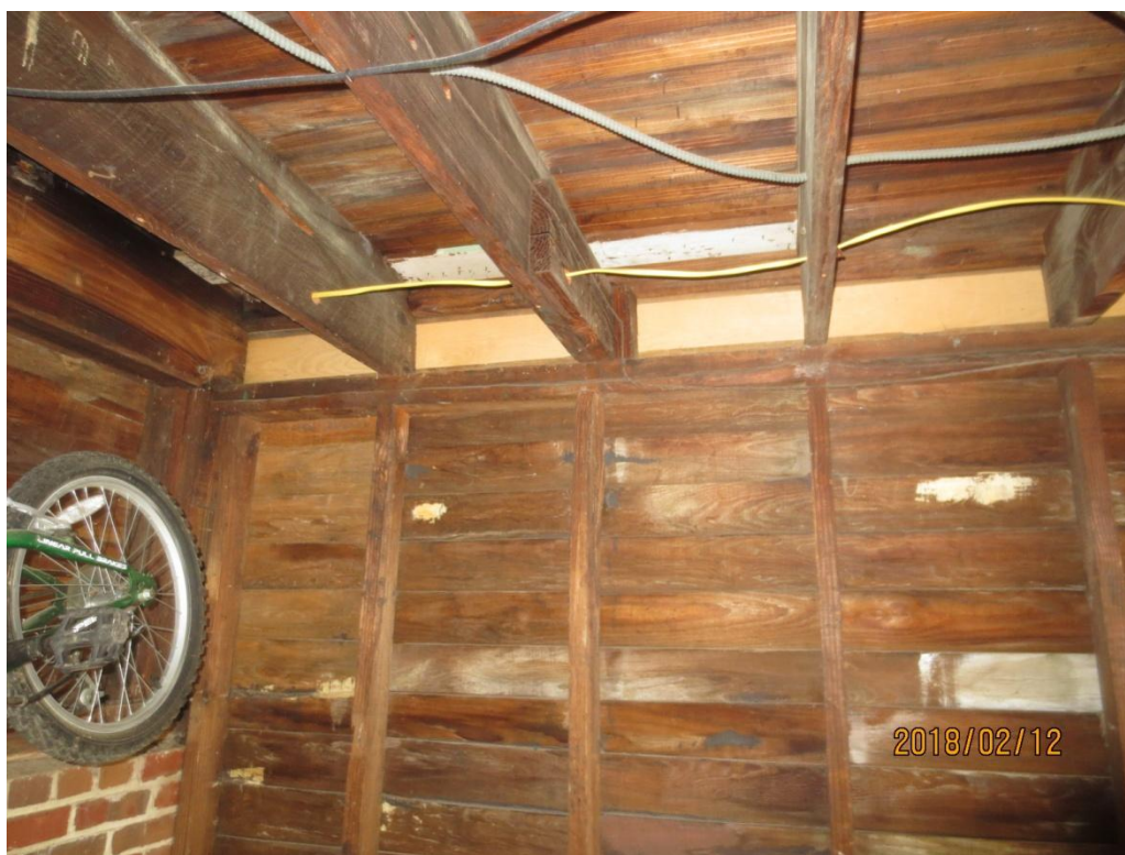
Damaged wall framing to be replaced
