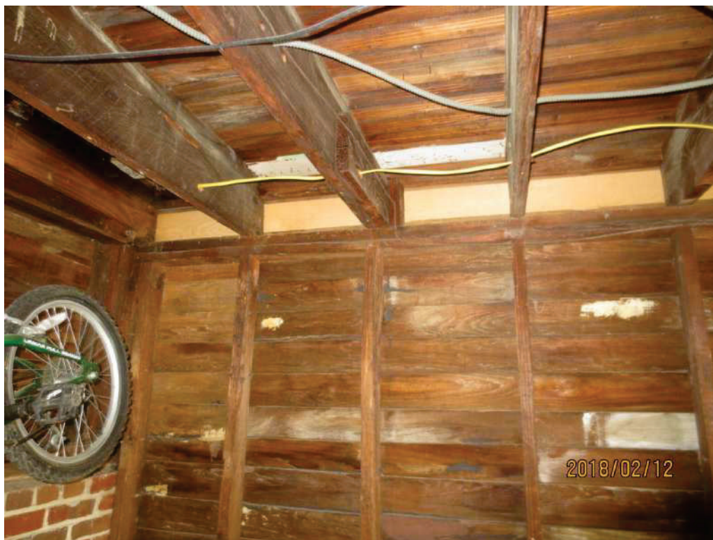
Damaged wall framing to be replaced
