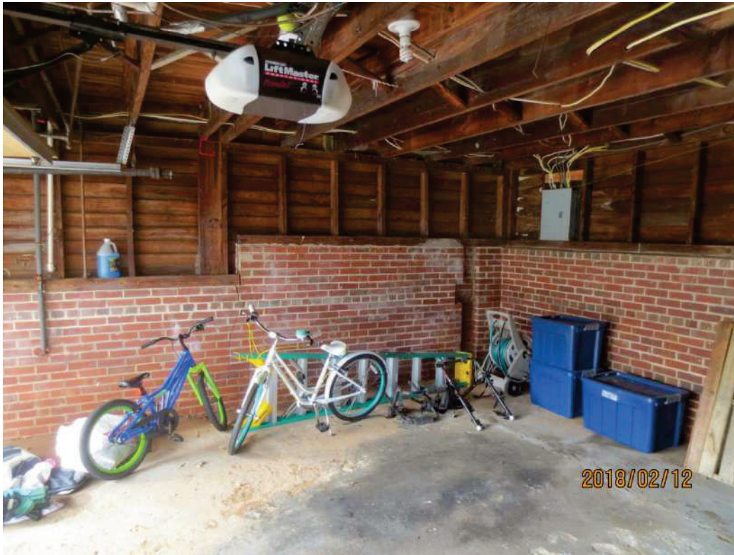
Left foundation wall and over-spans 2x12 joists
