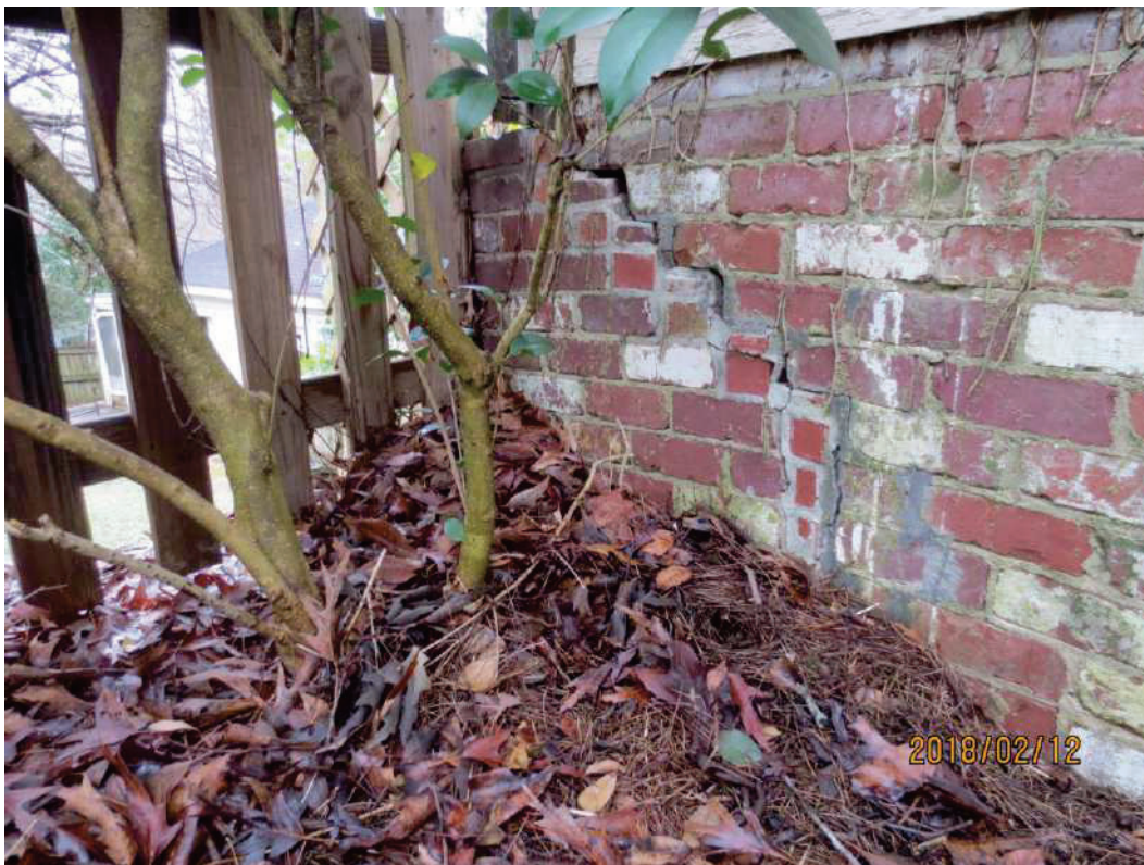
Rear addition corner settlement to be re-built with new footing and wall
