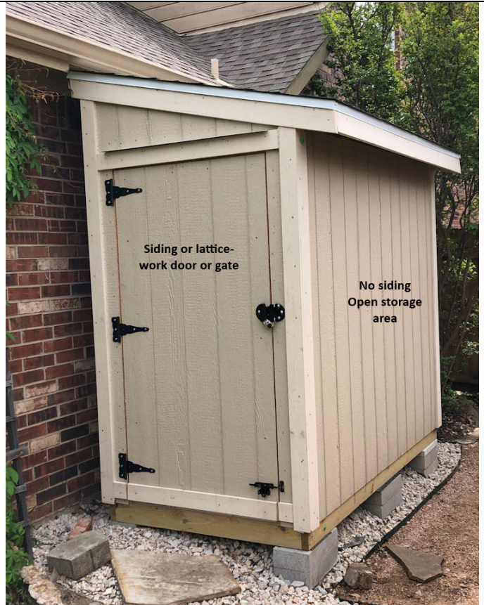
Figure 22. Example of construction of lean-to shed. Approximately 12' long and 3.5' wide. Lean-to roof to extend from and match the pitch of the existing garage roof. Clad in siding to match the gable siding of existing garage.
