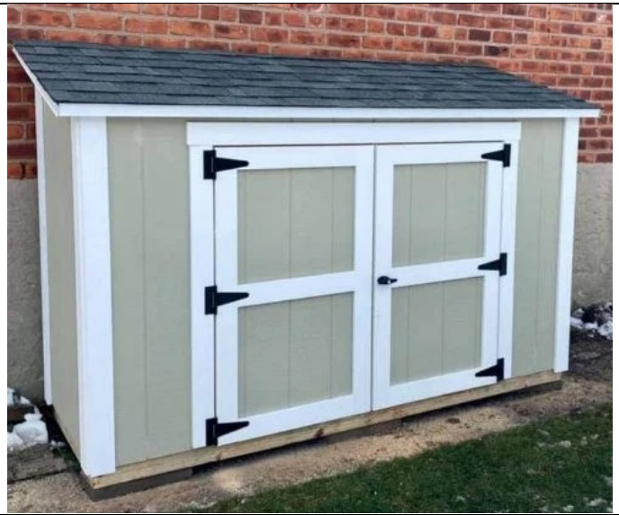
Figure 22. Example of construction of lean-to shed. Approximately 12' long and 3.5' wide. Lean-to roof to extend from and match the pitch of the existing garage roof. Clad in siding to match the gable siding of existing garage.
