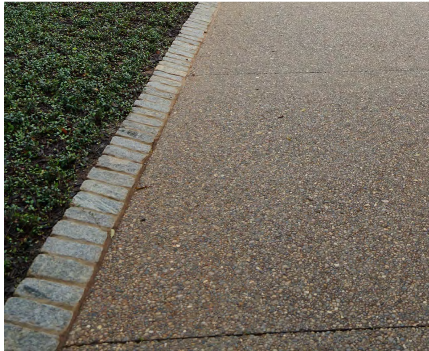
EXPOSED AGGREGATE MOTORCOURT WITH COBBLESTONE BORDER
