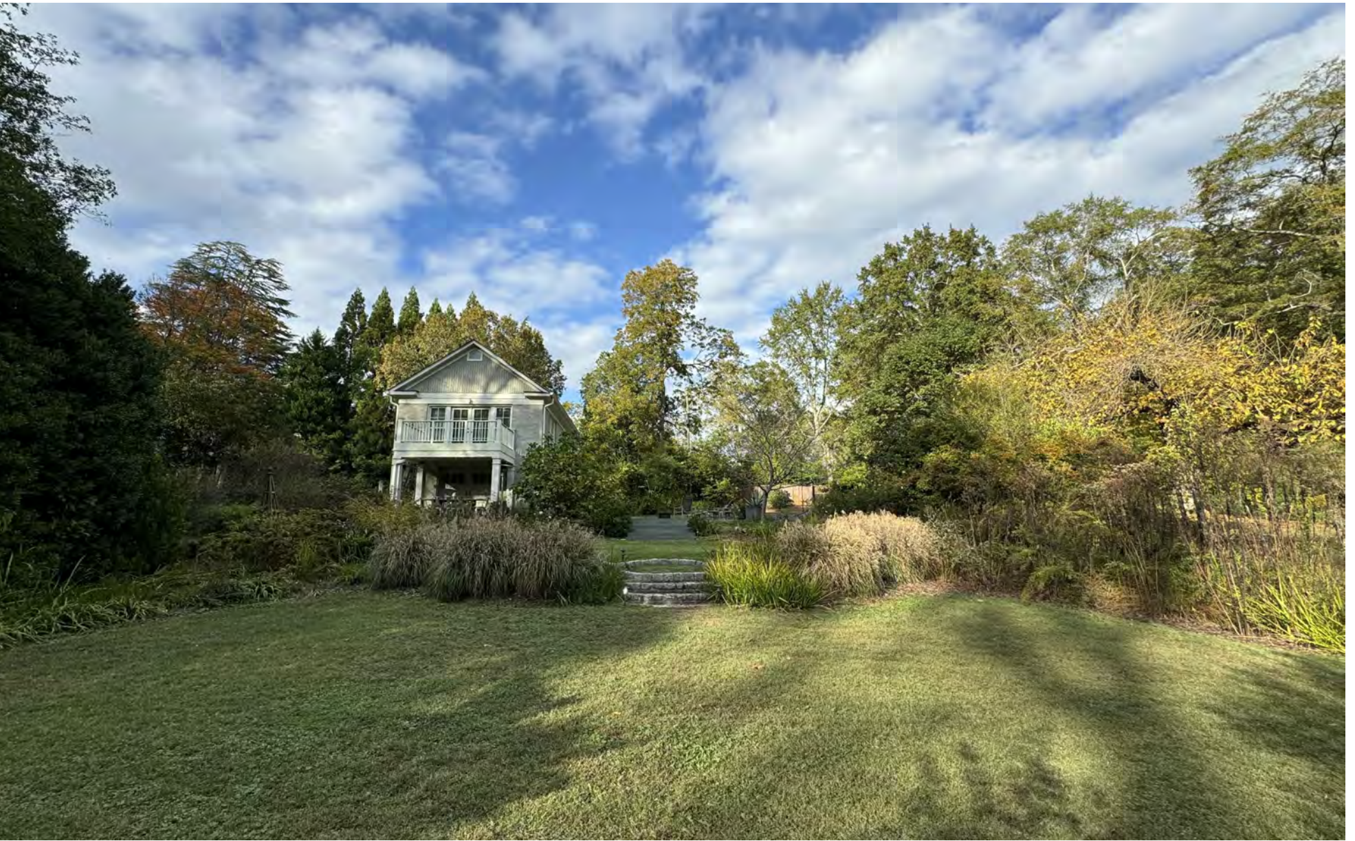
SOUTH SIDE OF EXISTING GARAGE / GUEST HOUSE
