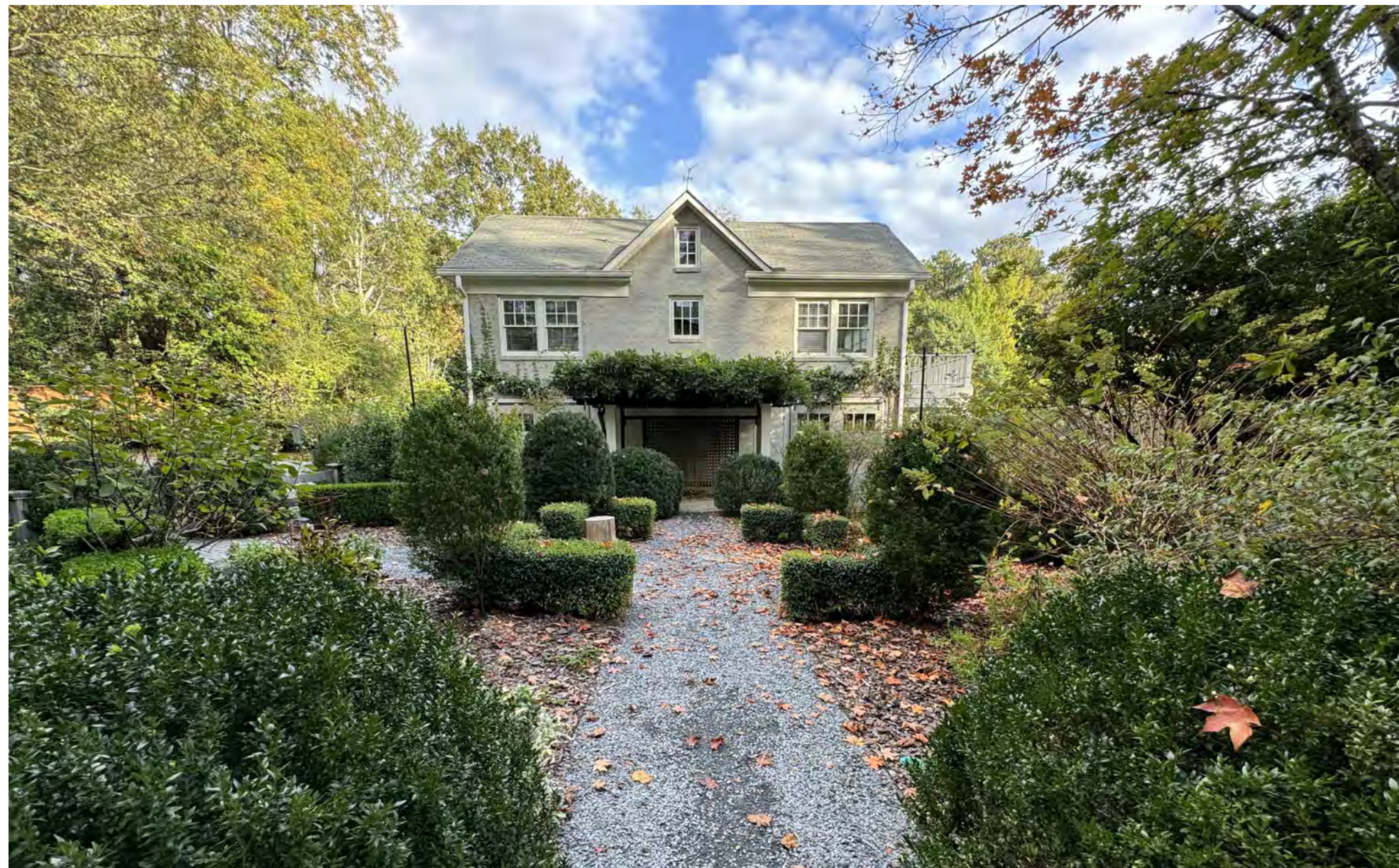
FRONT FACADE OF EXISTING GARAGE / GUEST HOUSE
