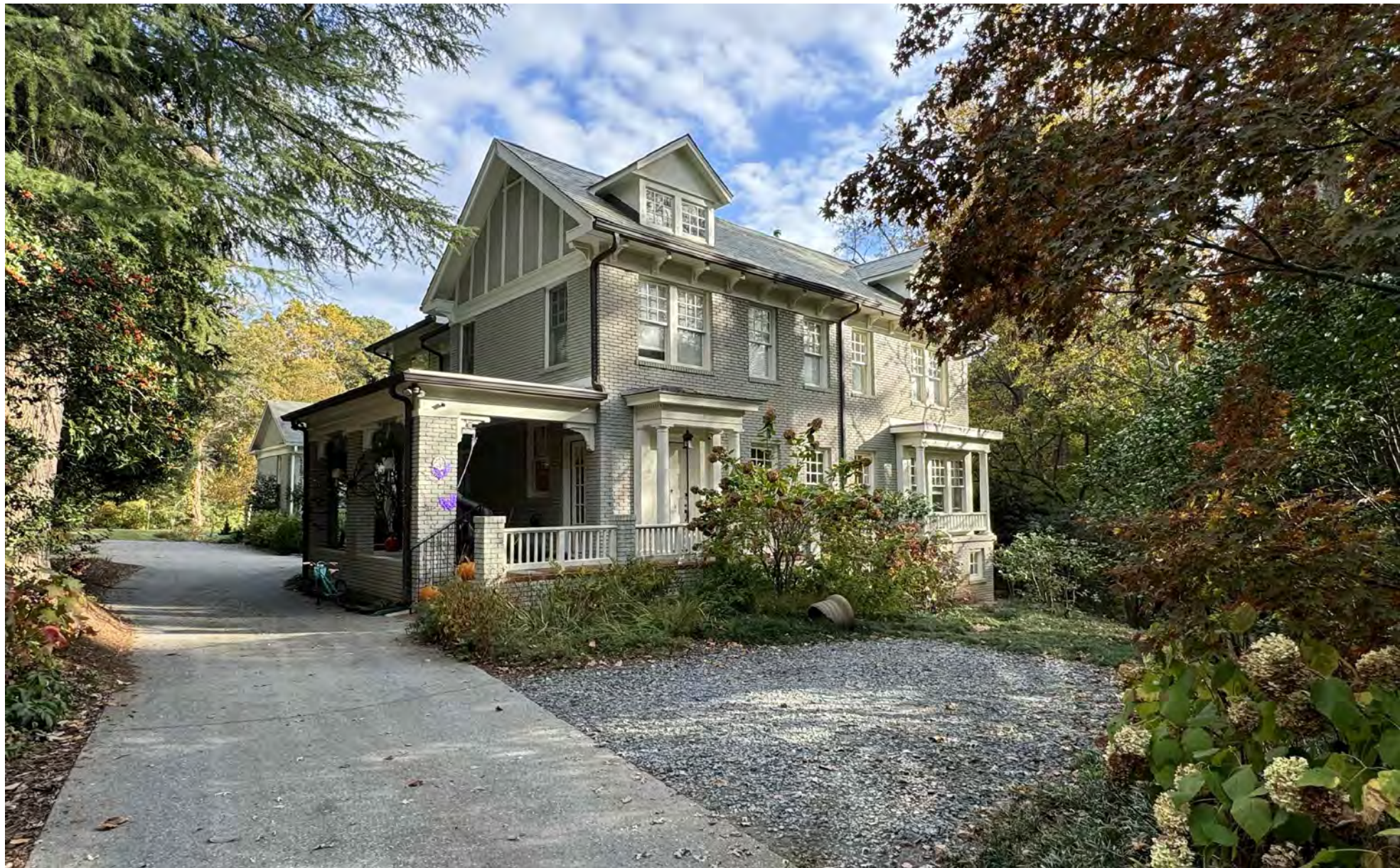
FRONT FACADE OF MAIN RESIDENCE
