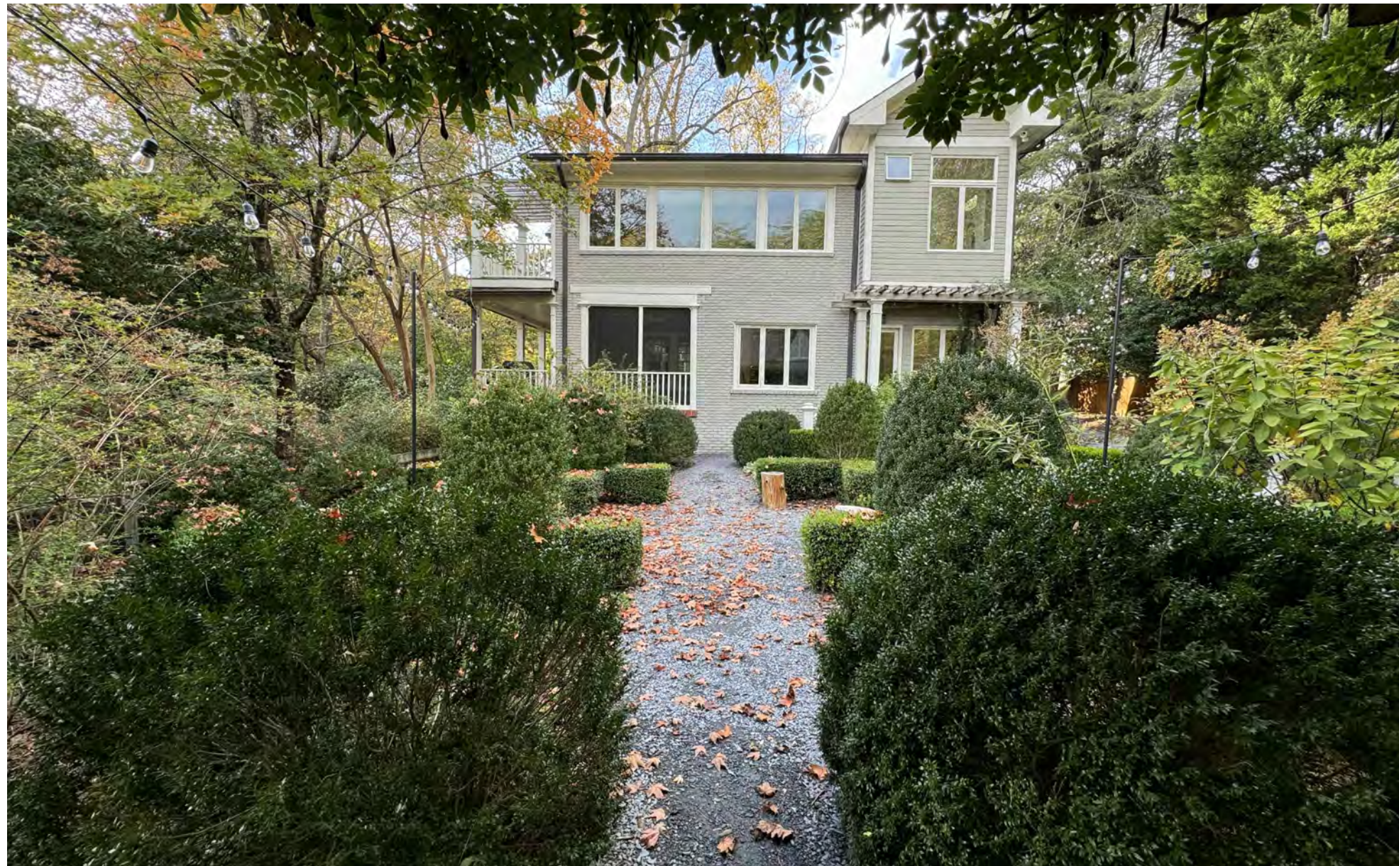
REAR FACADE OF MAIN RESIDENCE
