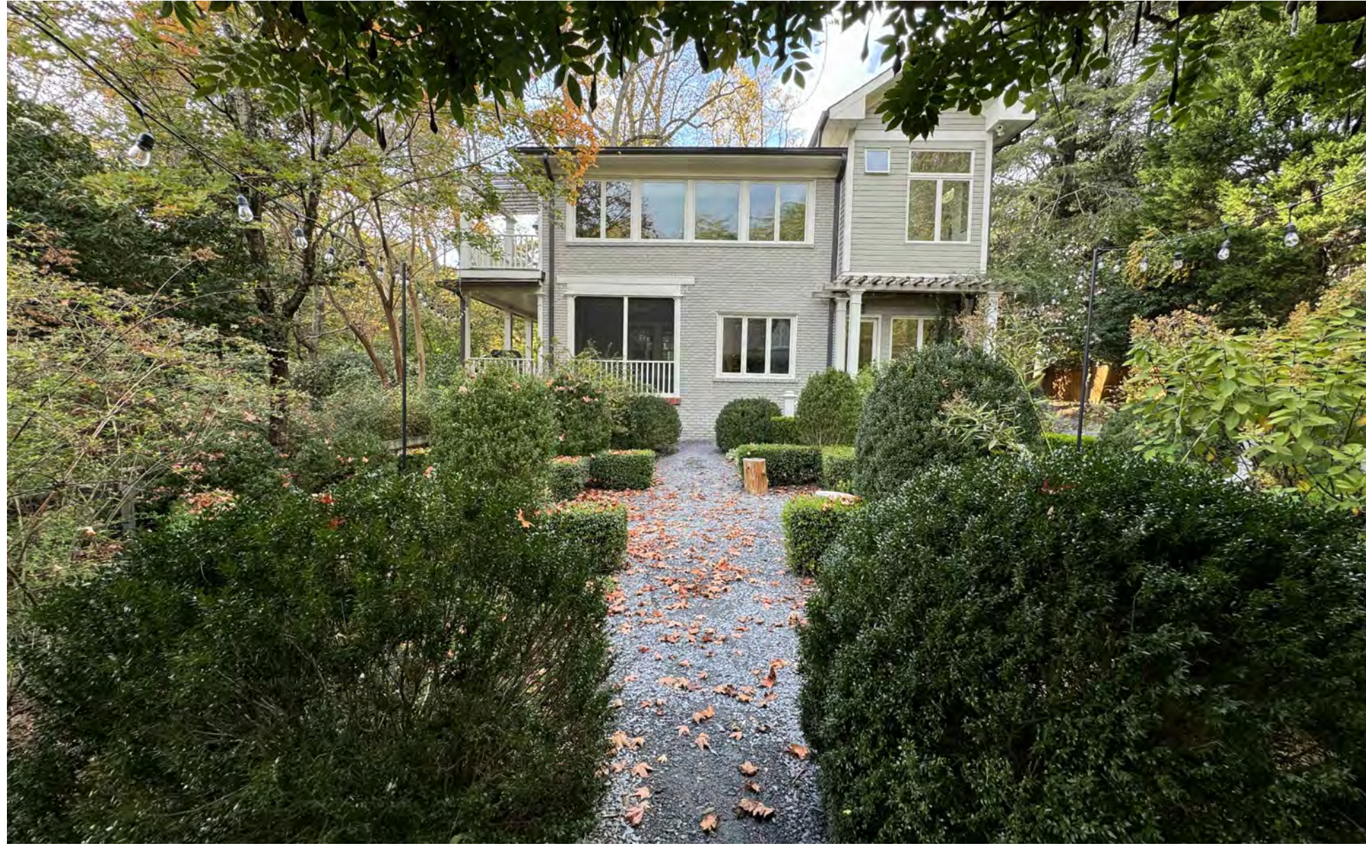
REAR FACADE OF MAIN RESIDENCE
