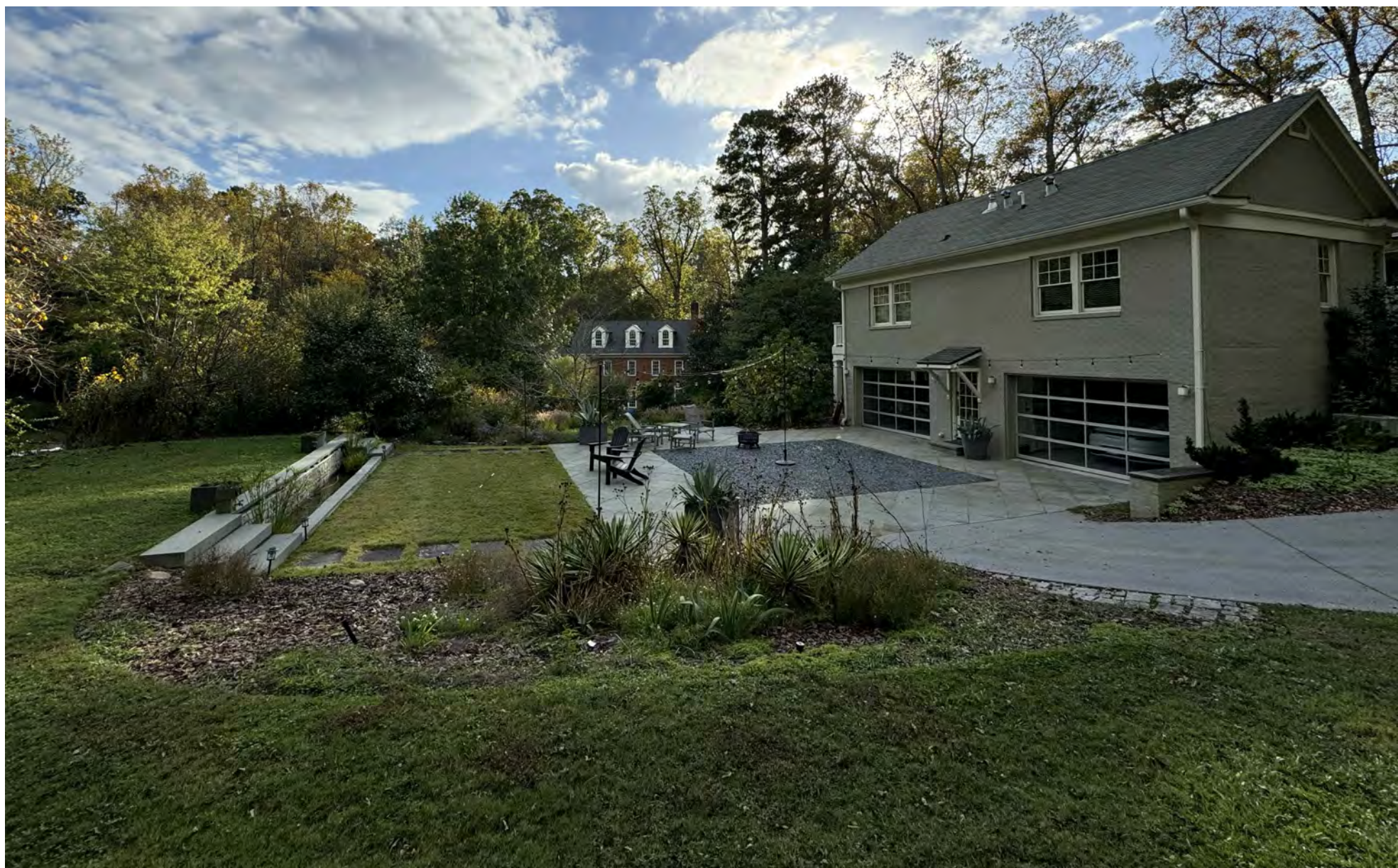
SIDE & REAR OF EXISTING GARAGE / GUEST HOUSE
