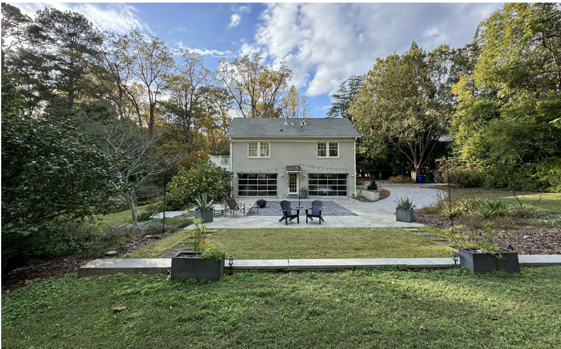
REAR FACADE OF EXISTING GARAGE / GUEST HOUSE
