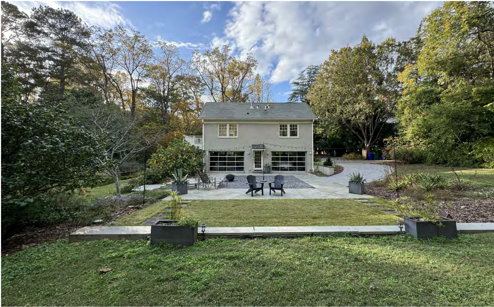
REAR FACADE OF EXISTING GARAGE / GUEST HOUSE
