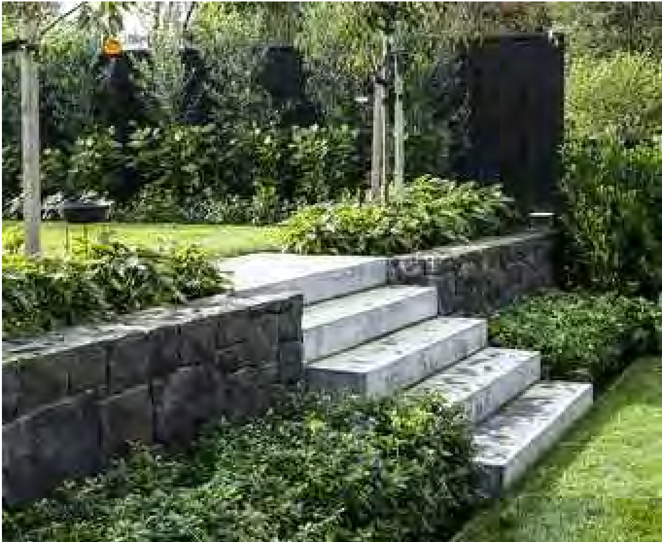
FIELDSTONE WALL WITH SLAB STEPS
